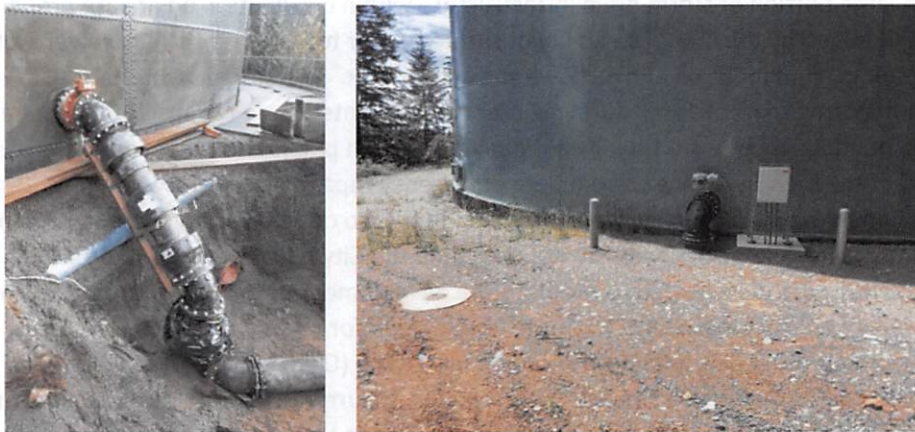
2018 Reservoir Seismic Valve Installation
