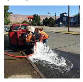
Occasionally main flushing causes water flowing from a tap to be discolored from stirred up sediment or milky white caused by tiny air bubbles. Although discolored water won't make you sick, you might want to flush the pipe by running the water for several minutes before drinking or washing.
