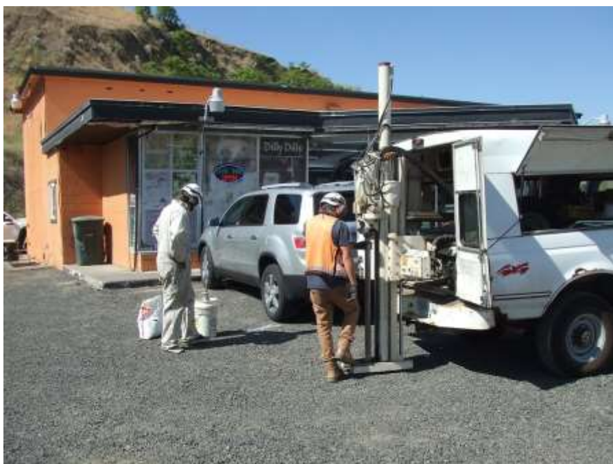
Photo 12. A view of the soil boring – B2.
