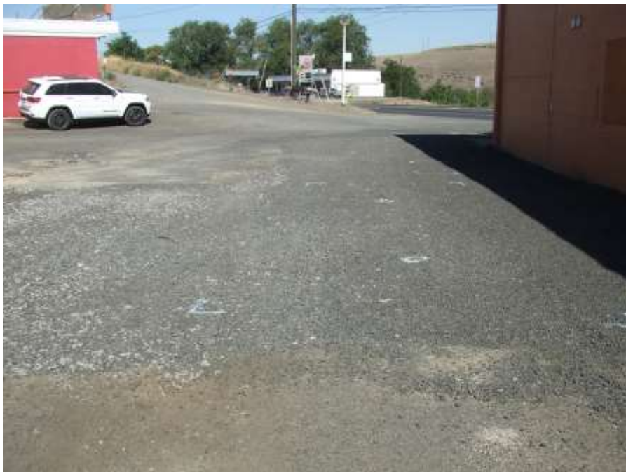
Photo 6. A view of the former USTs pad at the rear of the building looking west.
