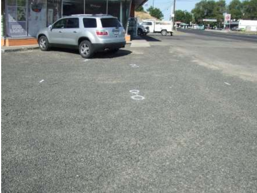
Photo 5. A view of the former USTs pad looking west.
