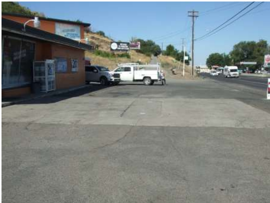
Photo 4. A view of the former pump island looking west.
