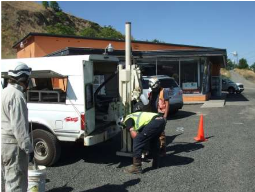
Photo 11. A view of the soil boring – B1.
