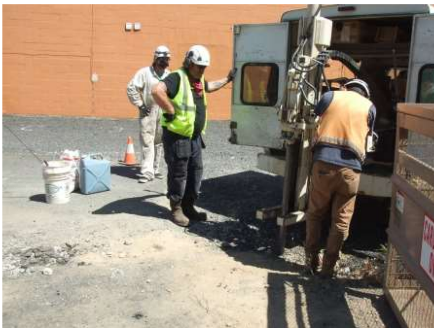
Photo 16. A view of the soil boring – B6.
