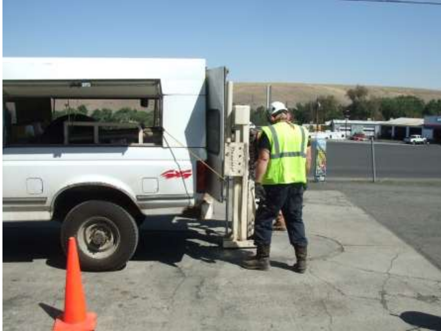
Photo 13. A view of the soil boring – B3.
