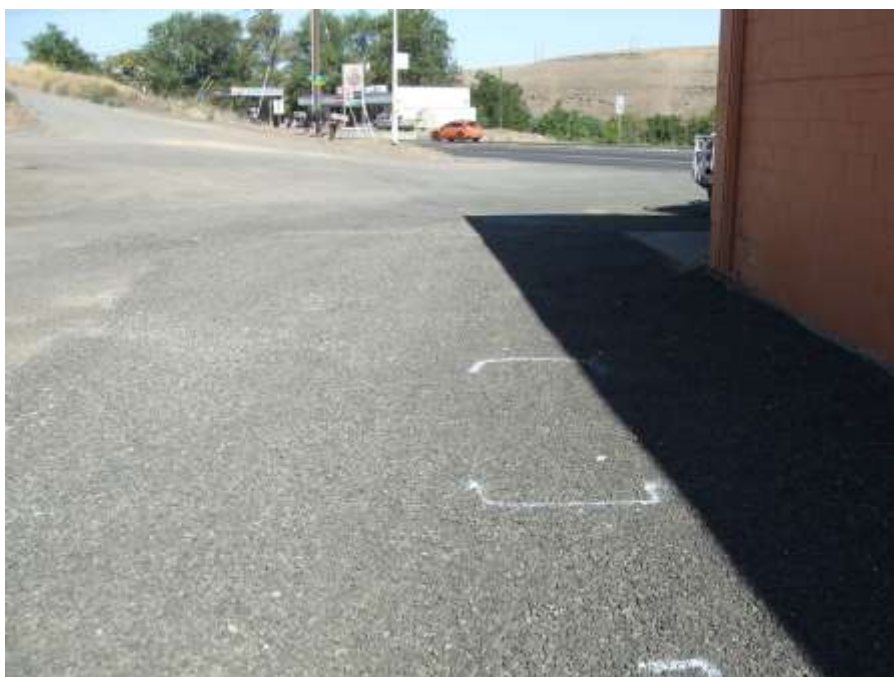
Photo 8. A view of the former waste oil UST pad looking west.
