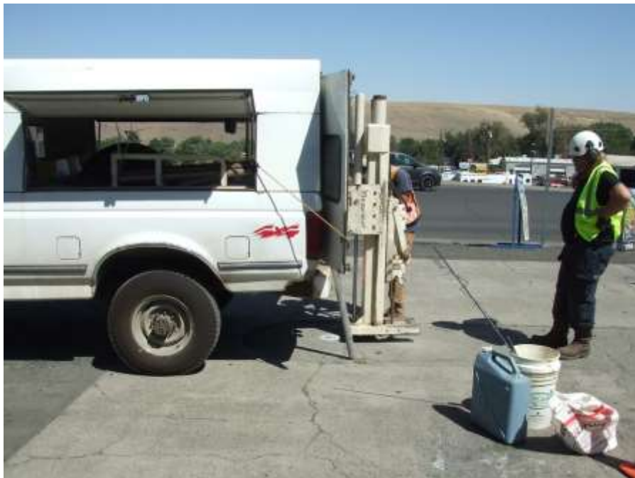
Photo 14. A view of the soil boring – B4.
