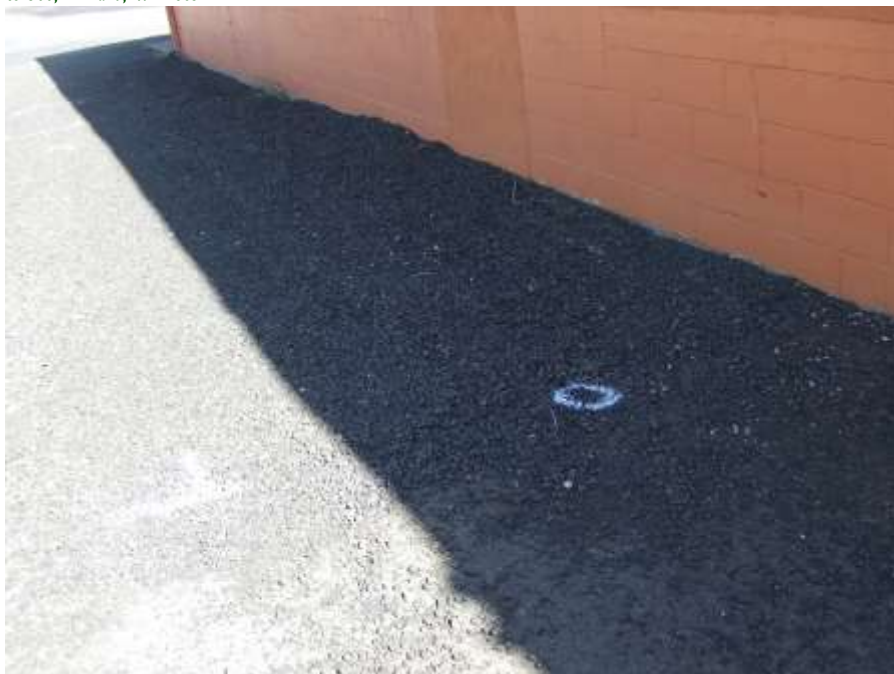
Photo 7. A view of the former heating oil location looking north.
