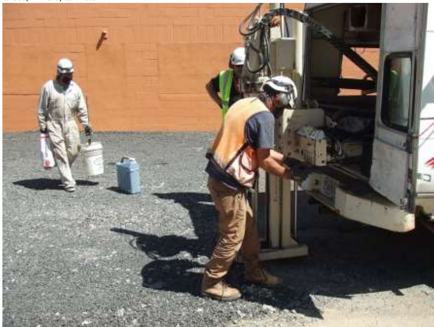
Photo 15. A view of the soil boring – B5.
