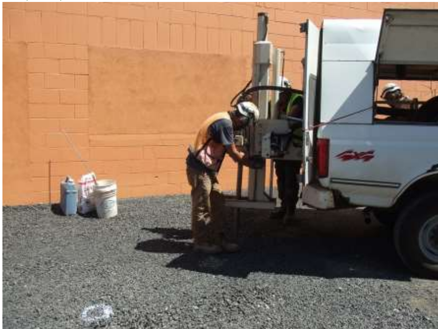
Photo 17. A view of the soil boring – B7.
