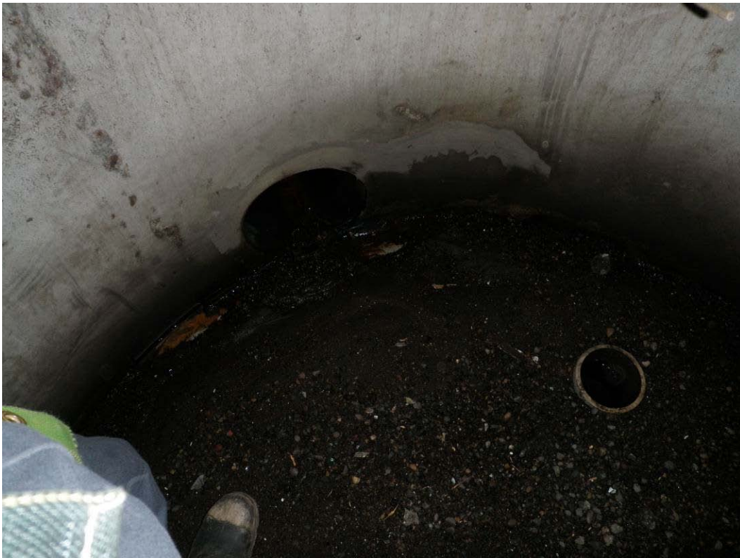
Photo 61 (September 8, 2010). Accumulated solids in ODOT manhole 4. Manhole is constructed as a sedimentation chamber.
