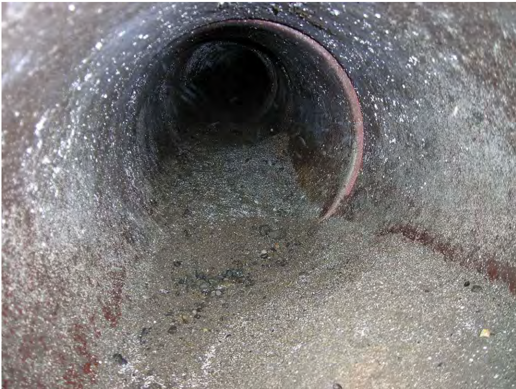
Photo 7 (June 26, 2008). 12-inch line entering manhole AAE569 from the east-southeast; view of solids sampled.
