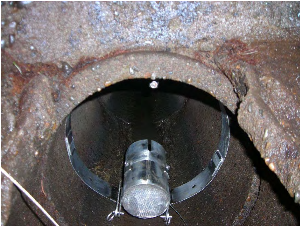
Photo 37 (February 2, 2010). SIFT© sediment trap installed in the 15-inch line entering manhole AAE513.
