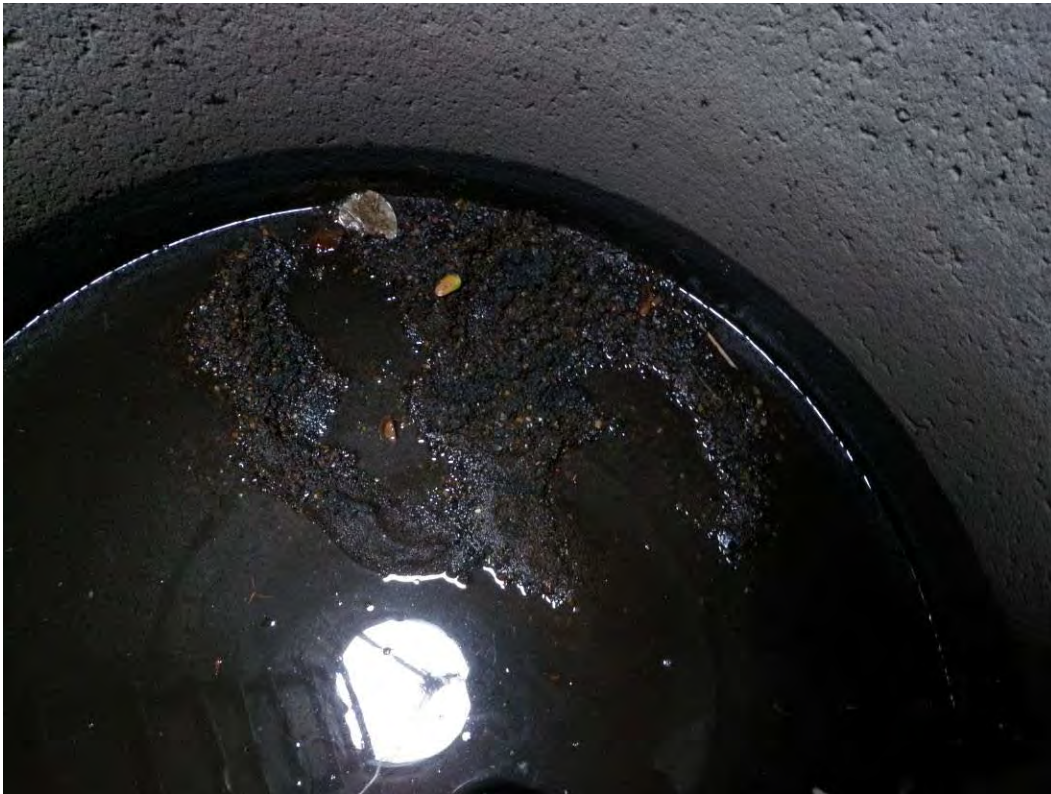
Photo 58 (September 7, 2010). Sediment and standing water inside ODOT manhole 2.
