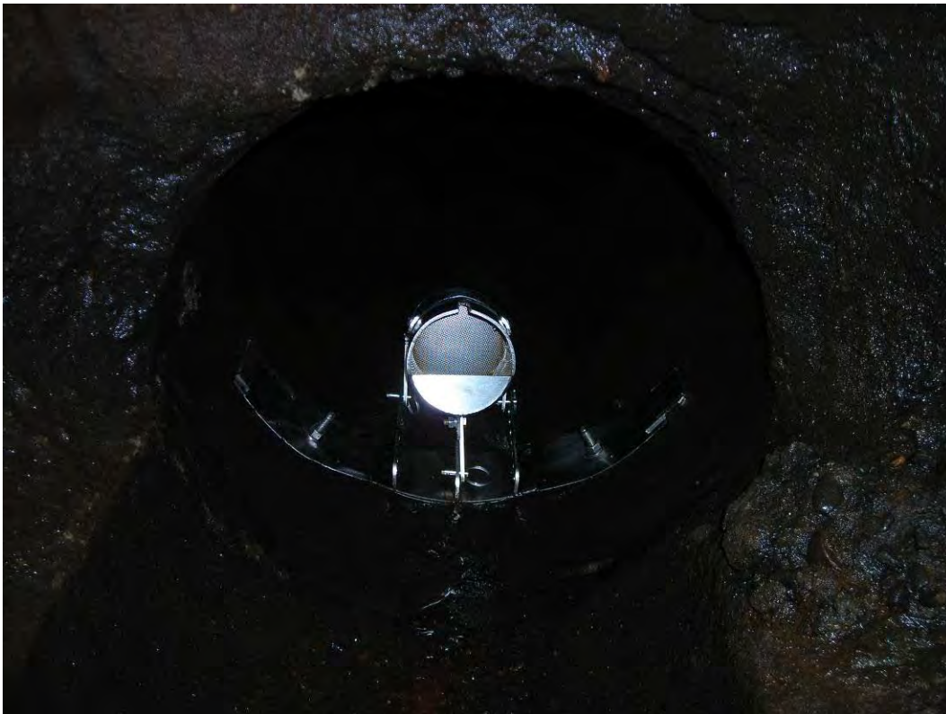
Photo 49 (February 2, 2010). SIFT© sediment trap installed in the 27-inch line exiting manhole AAE516.
