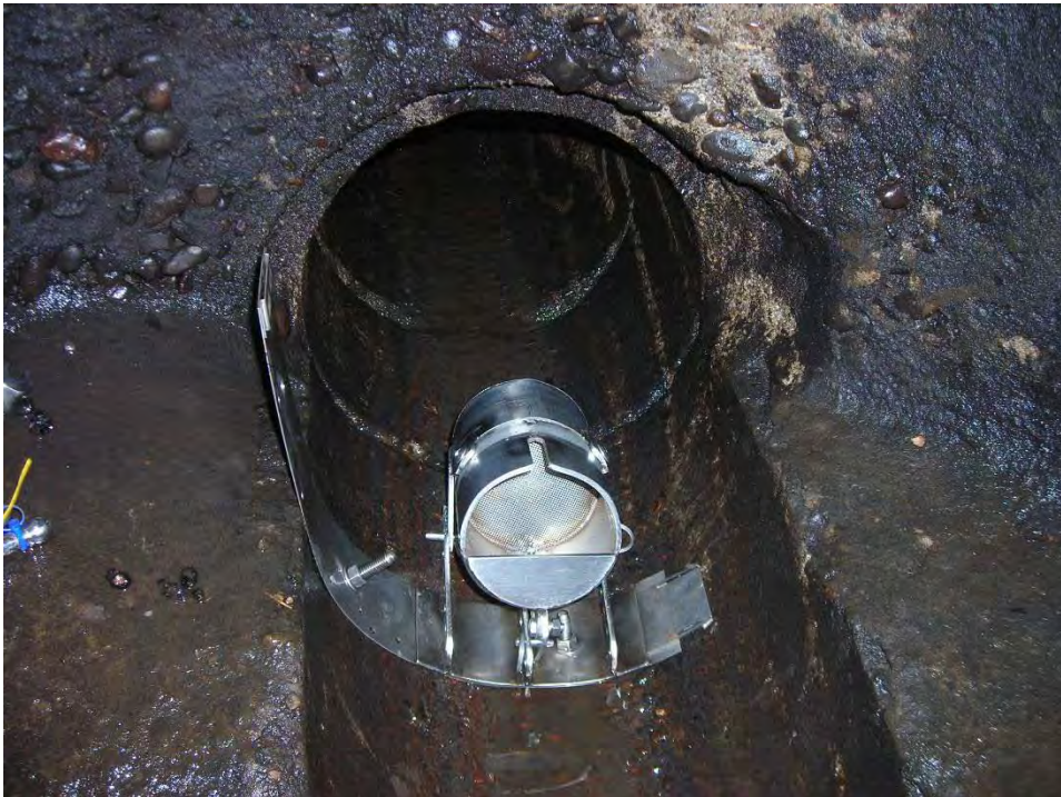
Photo 32 (February 2, 2010). SIFT© 1 sediment trap installed in the 12-inch line exiting manhole AAE498.
