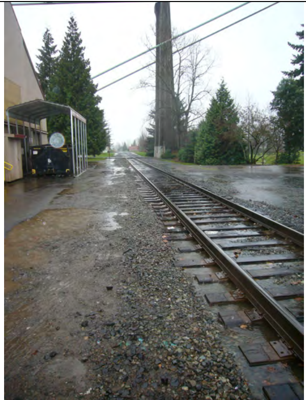
Looking south toward St Johns Bridge
