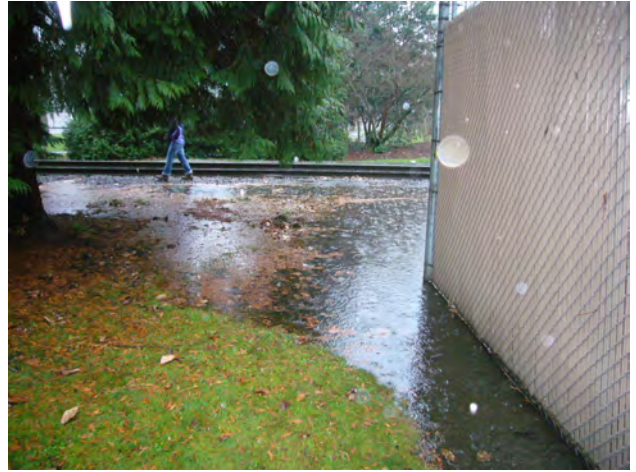
Ponded water near PIW storage area
