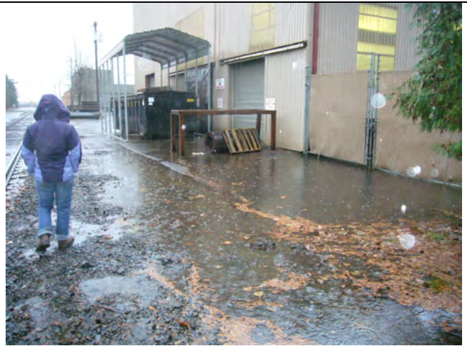
Ponding near PIW scrap storage area
