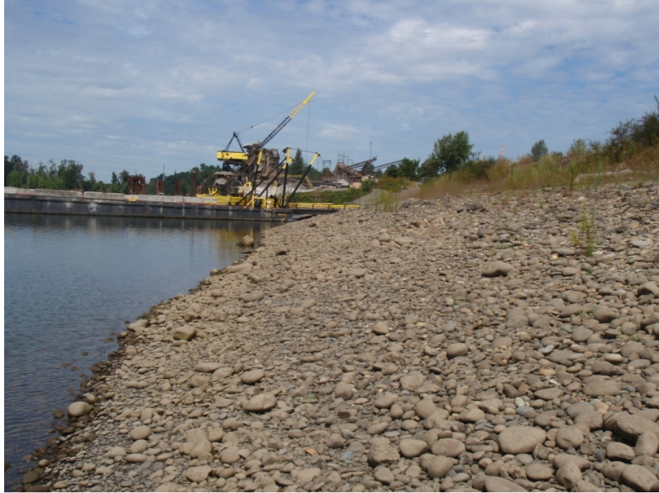
REMEDIAL ACTION SUB-AREA A2-2. FACING NORTH
