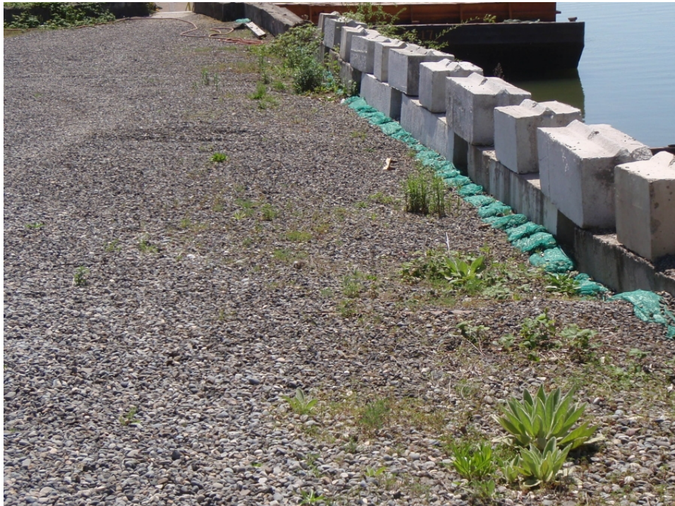
REMEDIAL ACTION SUB-AREA A2-1. ECOLOGY BLOCKS AND BIOFILTER BAGS, FACING SOUTH
