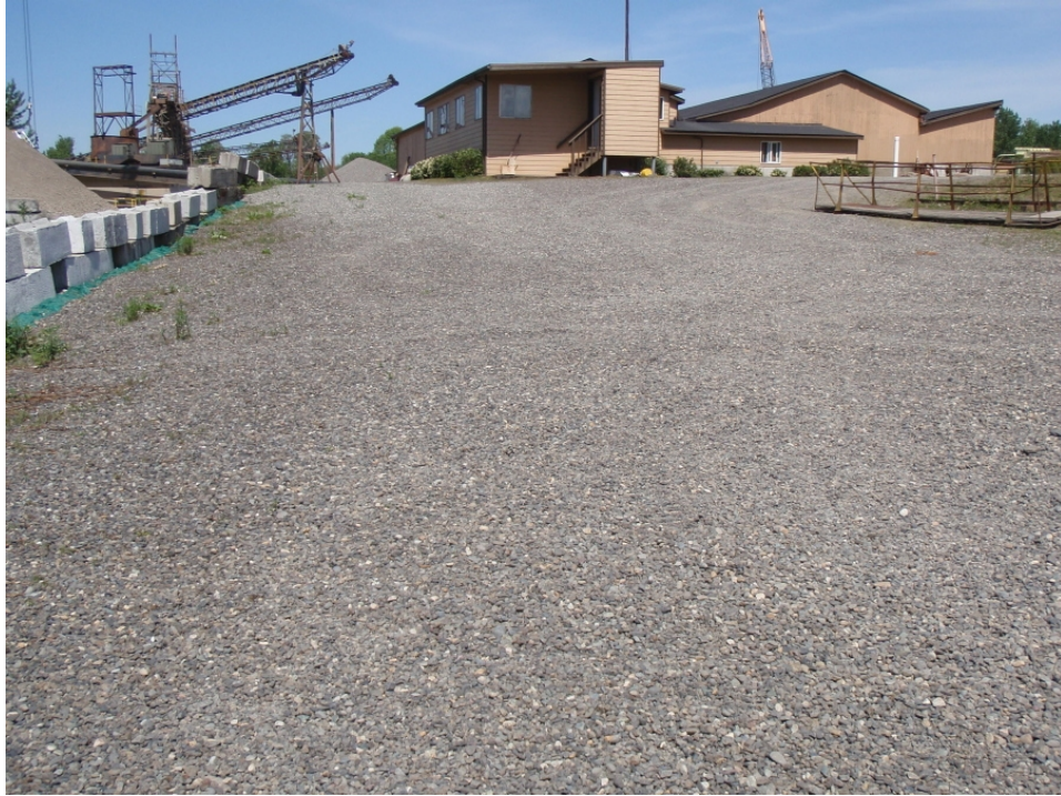
REMEDIAL ACTION SUB-AREA A2-1. FACING NORTH
