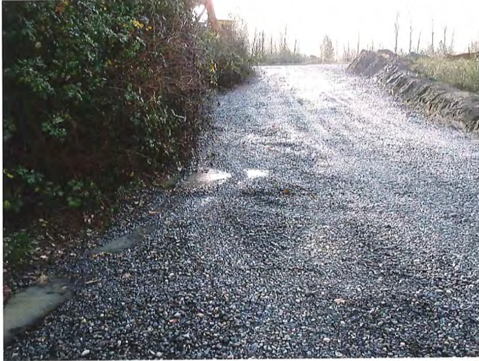
REMEDIAL ACTION SUB-AREA A2-3. DURING RAIN EVENT
