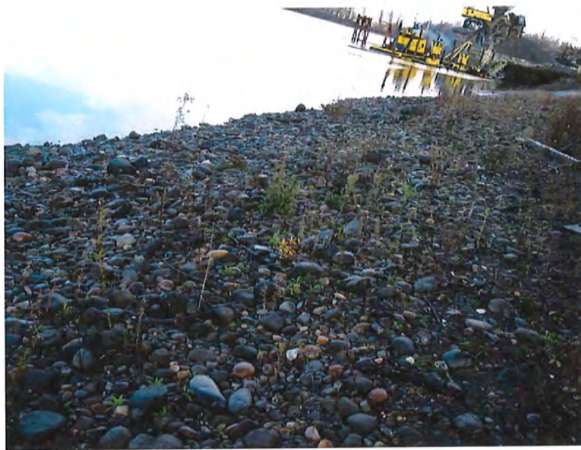
REMEDIAL ACTION SUB-AREA A2-2. DURING LOW WATER, FACING NORTH
