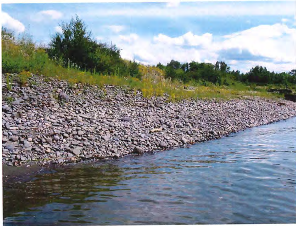
REMEDIAL ACTION SUB-AREA A2-2. FACING SOUTHEAST
