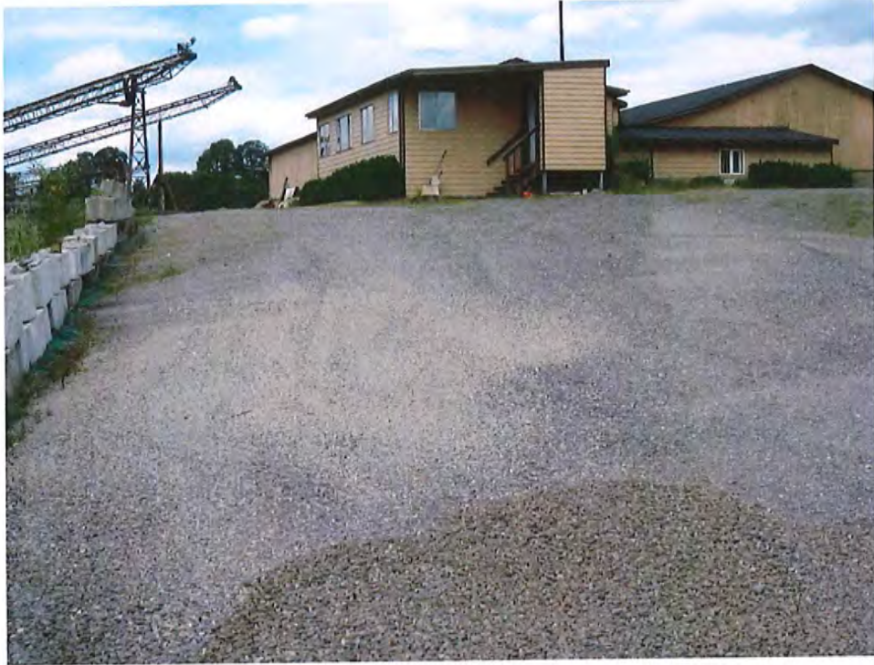
REMEDIAL ACTION SUB-AREA A2-1. FACING NORTH
