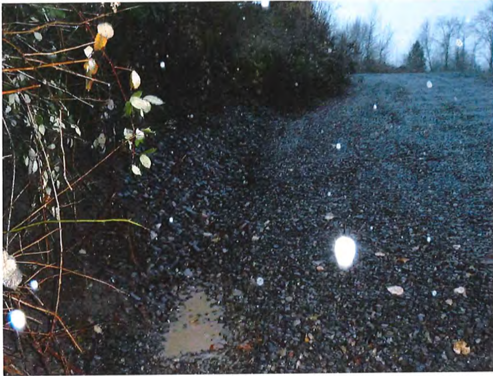
REMEDIAL ACTION SUB-AREA A2-3. DURING RAIN EVENT
