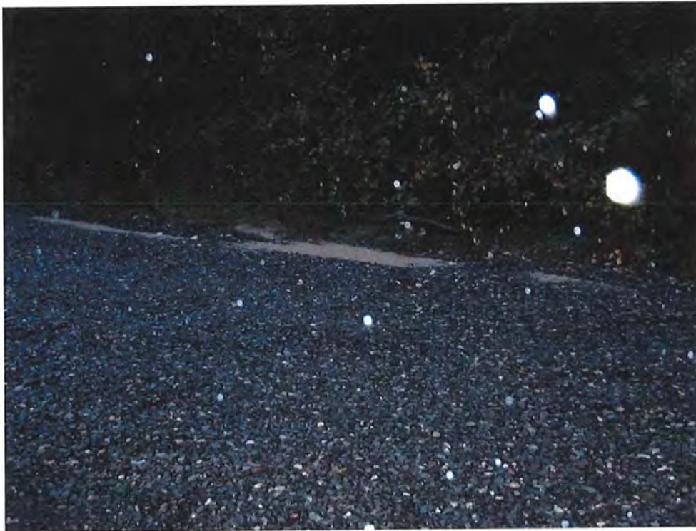
REMEDIAL ACTION SUB-AREA A2-3, DURING RAIN EVENT
