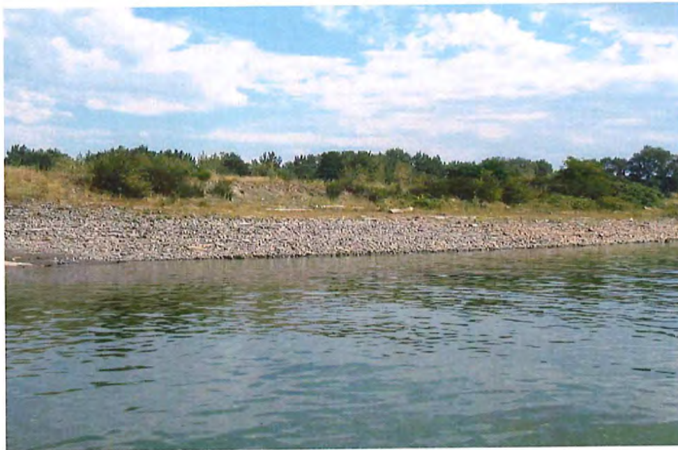
REMEDIAL ACTION SUB-AREA A2-2. DURING LOW WATER. FACING SOUTH
