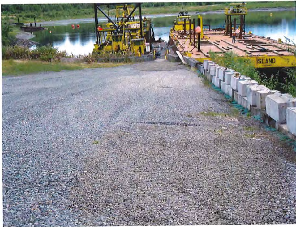
REMEDIAL ACTION SUB-AREA A2-1.ECOLOGY BLOCKS AND BIOFILTER BAGS FACING SOUTH
