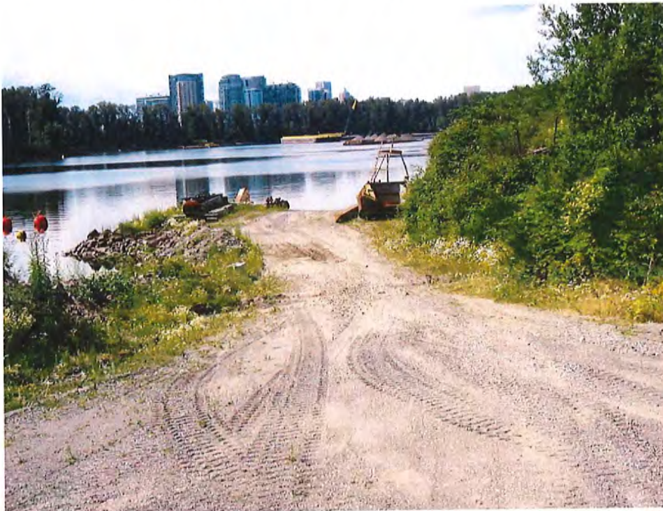
REMEDIAL ACTION SUB-AREA A2-3, FACING NORTHWEST
