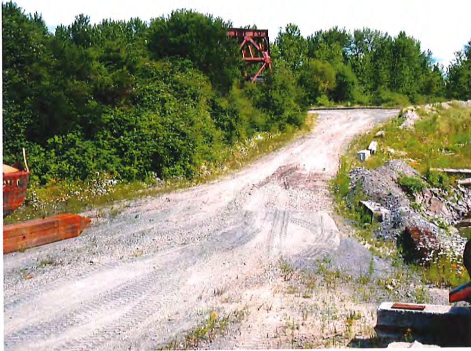
REMEDIAL ACTION SUB-AREA A2-3. FACING SOUTHEAST
