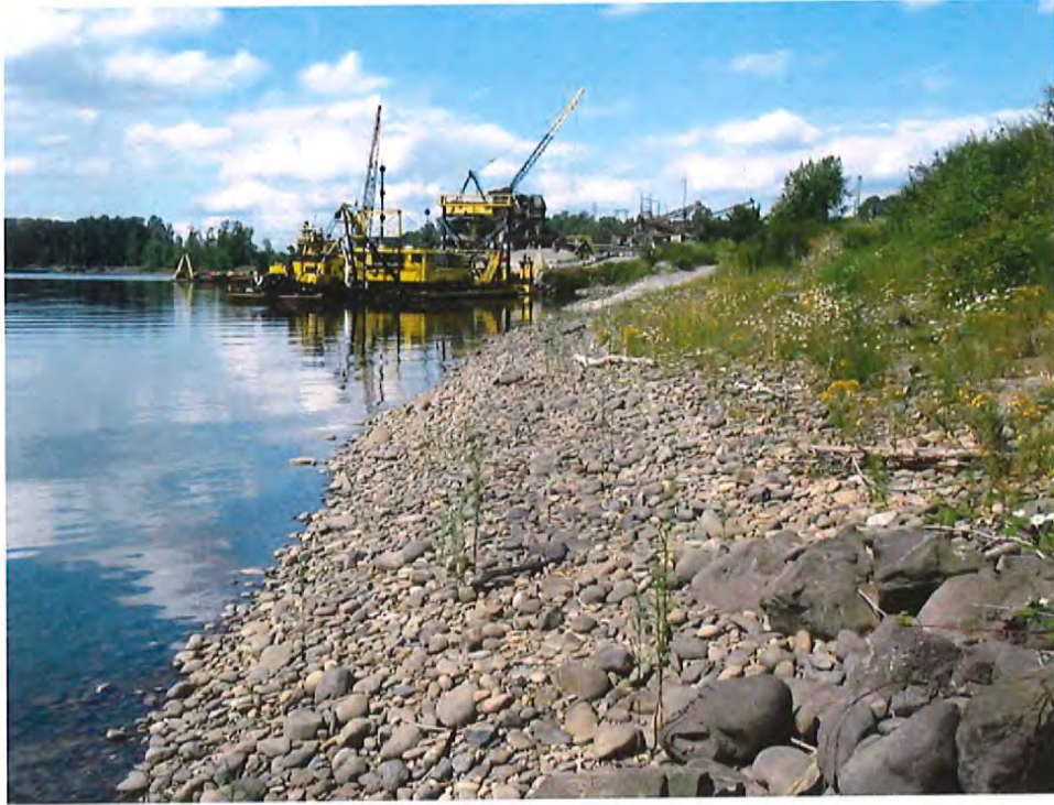
REMEDIAL ACTION SUB-AREA A2-2. FACING NORTH
