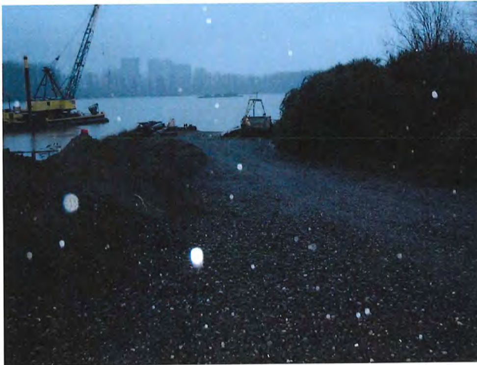
REMEDIAL ACTION SUB-AREA A2-3, DURING RAIN EVENT
