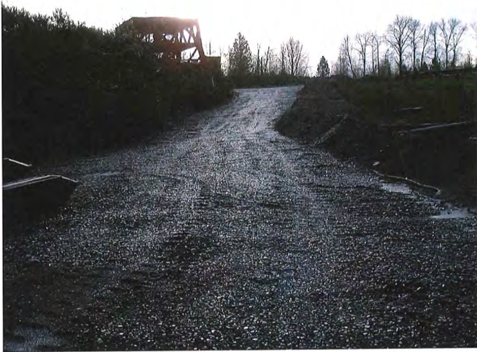
REMEDIAL ACTION SUB-AREA A2-3. DURING RAIN EVENT
