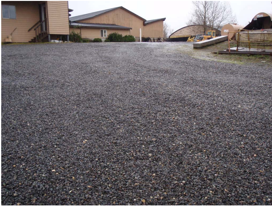
REMEDIAL ACTION SUB-AREA A2-1. PHOTOGRAPH TAKEN MARCH 21, 2012 FACING NORTH.
