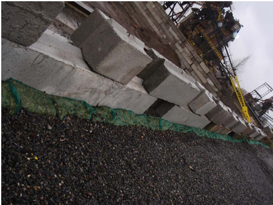
REMEDIAL ACTION SUB-AREA A2-1. ECOLOGY BLOCK AND BIOFILTER BAGS. PHOTOGRAPH TAKEN MARCH 21, 2012 FACING NORTH.
