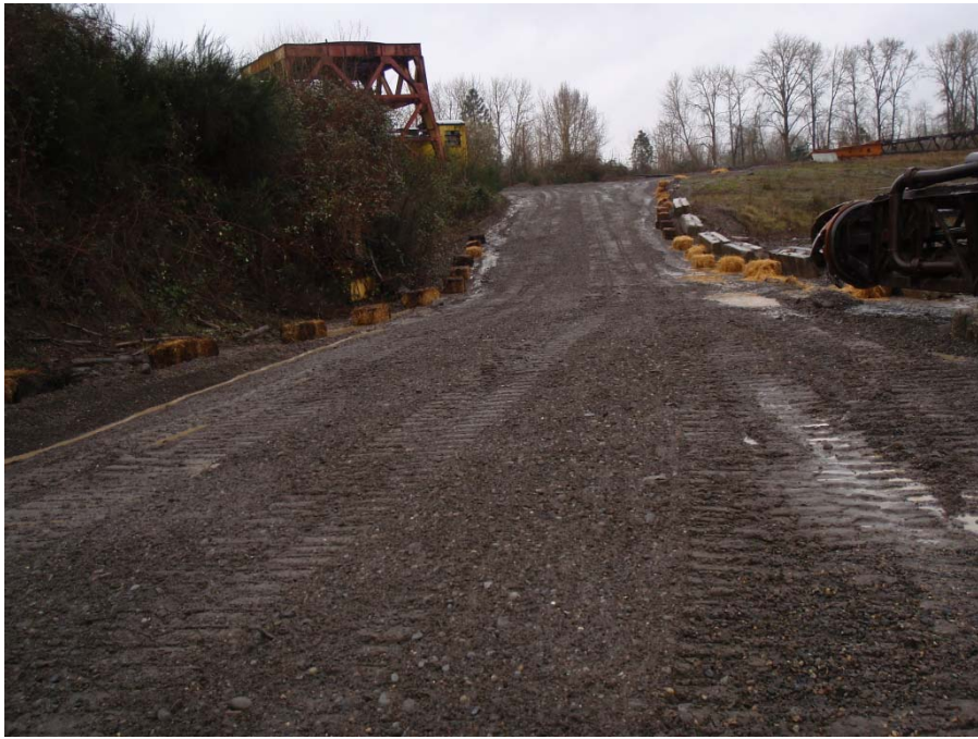
REMEDIAL ACTION SUB-AREA A2-3. PHOTOGRAPH TAKEN MARCH 21, 2012 FACING SOUTHEAST.
