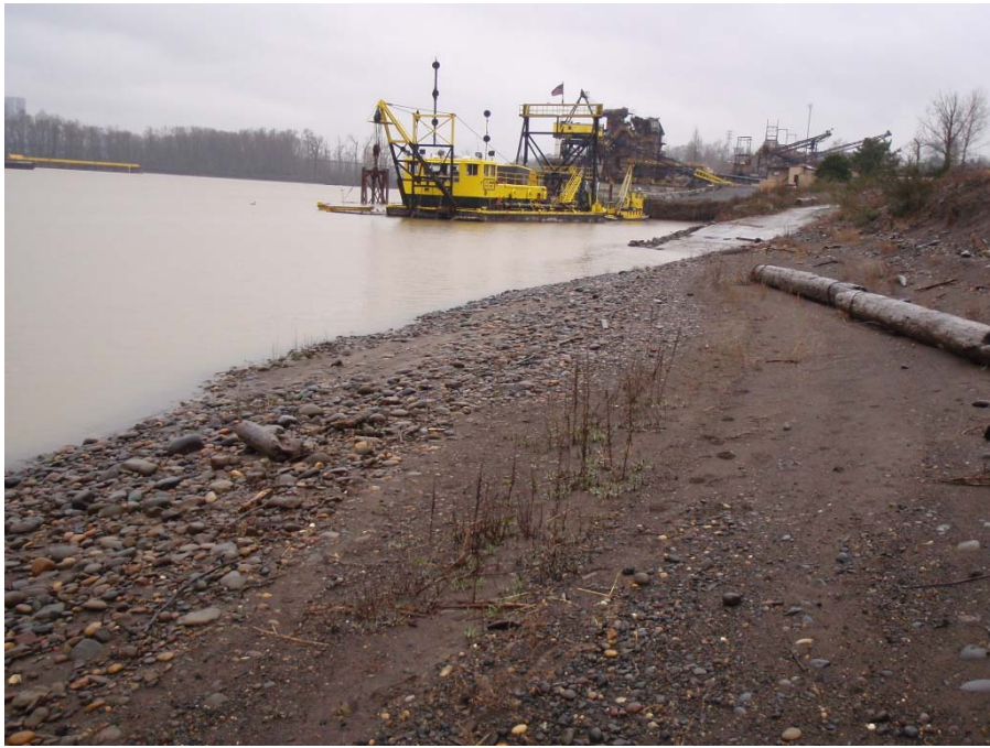
REMEDIAL ACTION SUB-AREA A2-2. PHOTOGRAPH TAKEN MARCH 21, 2012 FACING NORTH.
