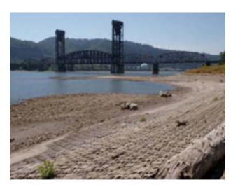
Figure 2. Exposed ACB and sand cap armoring at the McCormick & Baxter site.
