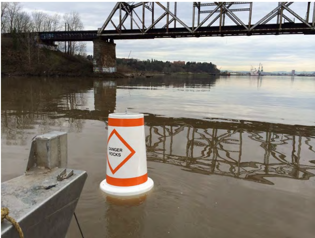
Photograph 3 – Buoy number 4 replacement.
