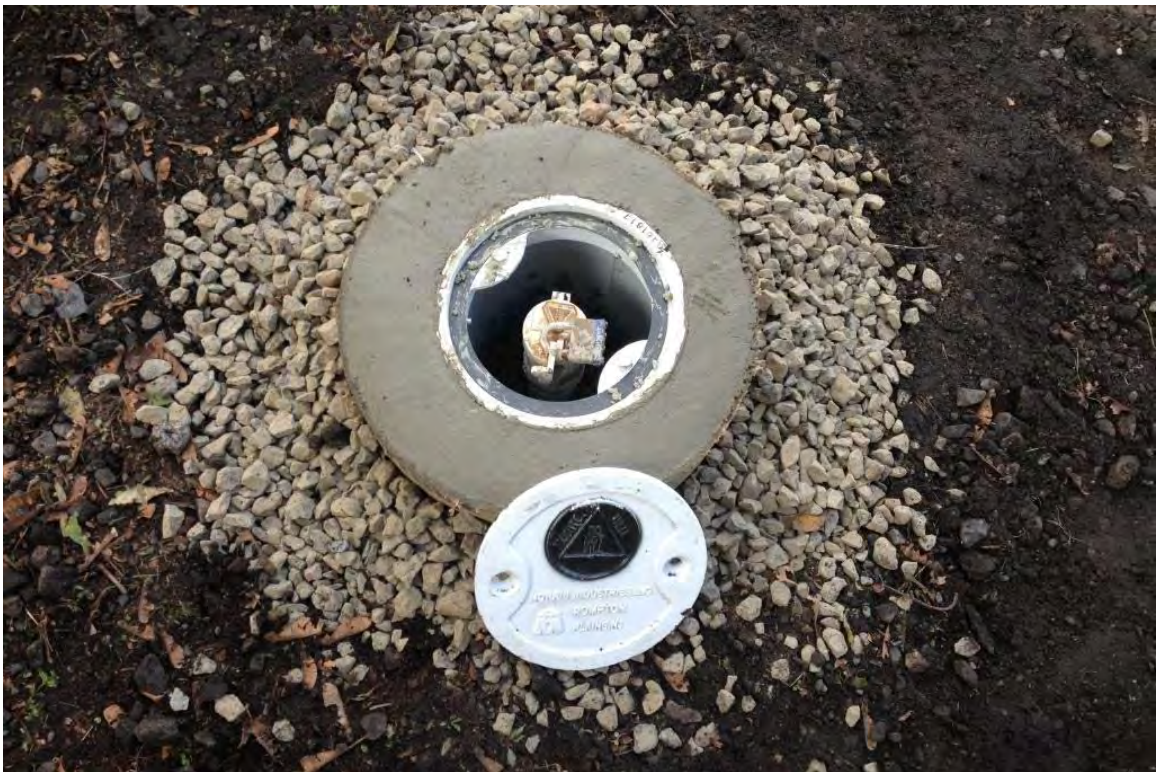
Photograph 9 - MW-58 well cluster repairs completed in 2013 without making modifications to the existing well casing heights.
