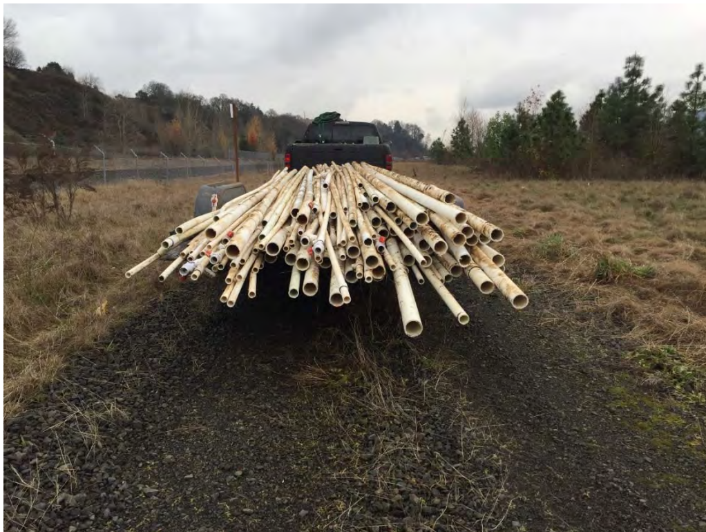
Photograph 11 – 2015 irrigation system decommissioning.
