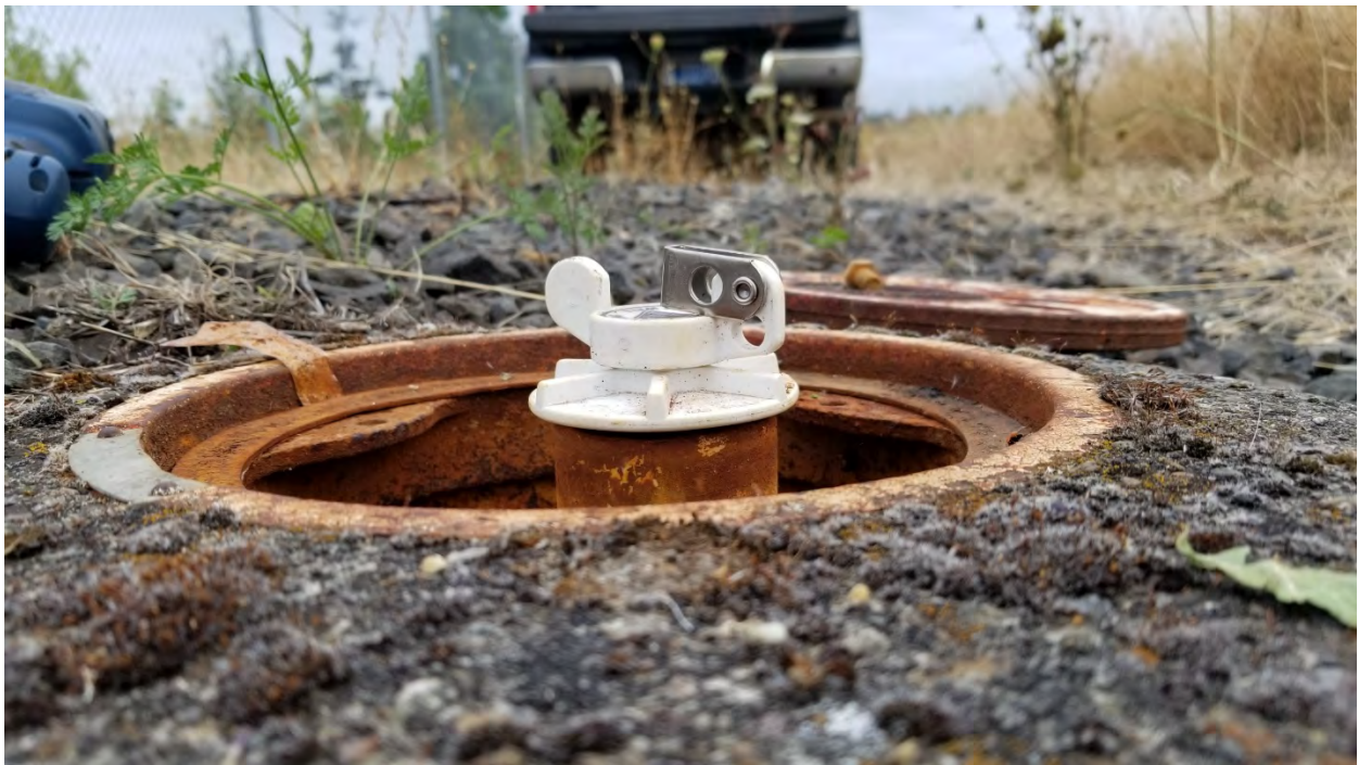
Photo 8: Well cap and casing for MW-59s protruding above the rim of the well box in the perimeter road.
