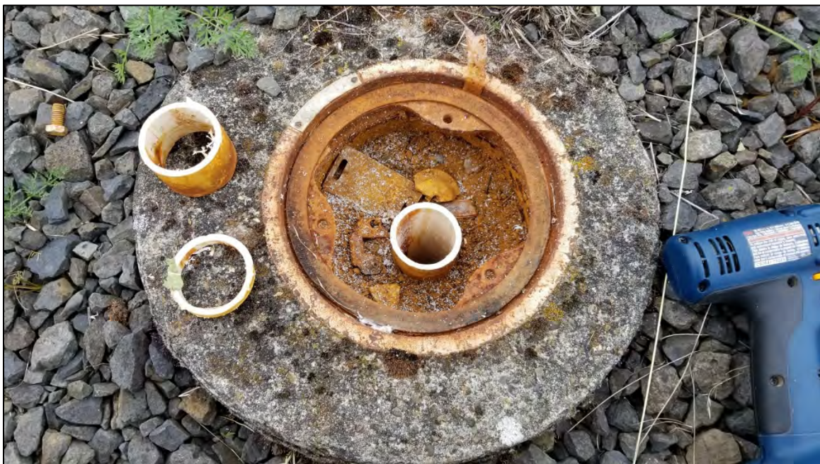
Photograph 13: Trimming MW-59s well casing to maintain well box lid functionality due to subsided well box, August 2019.
