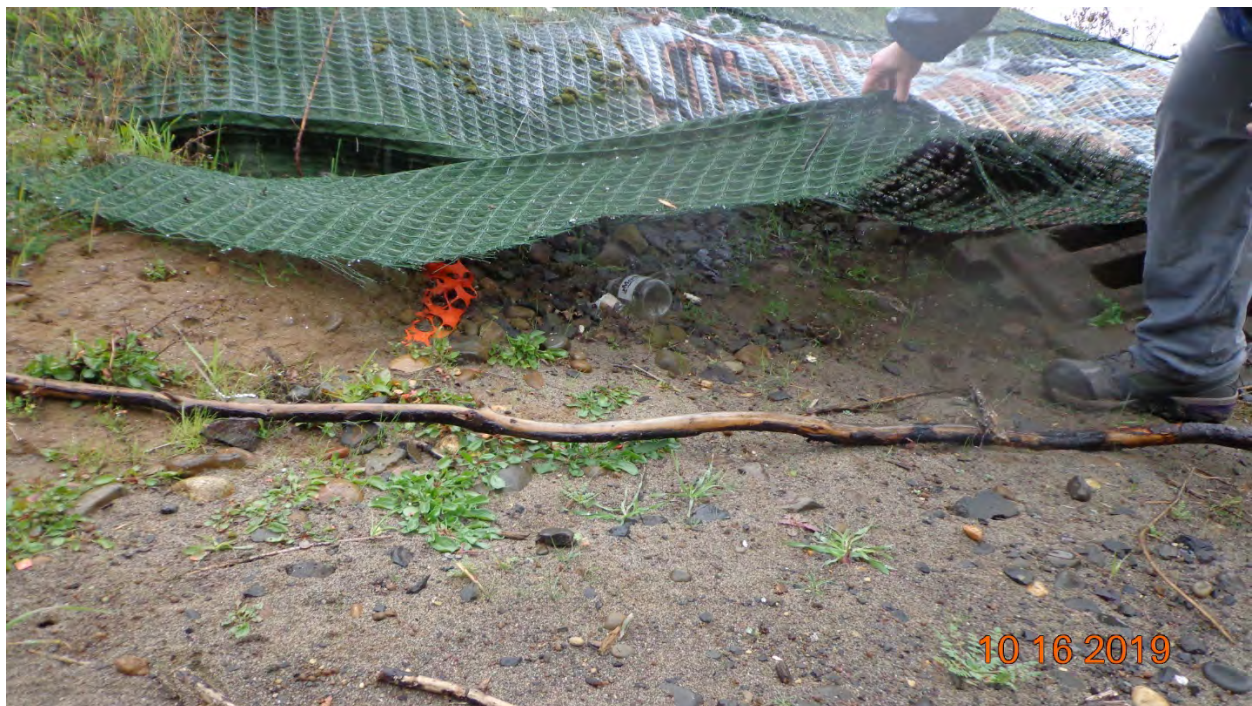
Photo 2: View of depression under TRM where sand appears to have washed out from under the corner of the mat.
