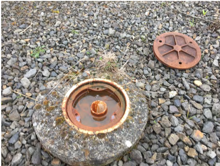
Photo 6 –View of the inner casing protruding past the monument in MW-59s.
