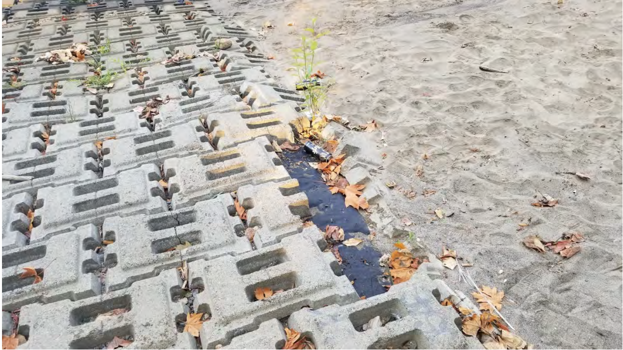
Photograph 1: Buckling and sagging of the ACB border on the eastern edge of the Willamette Cove ACB.
