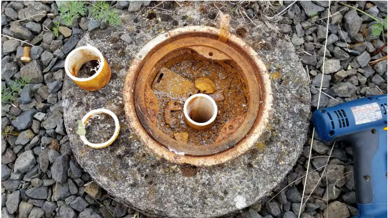
Photo 9: MW-59s well casing after removal of 3 inches using a power drill attached internal PVC pipe cutter.
