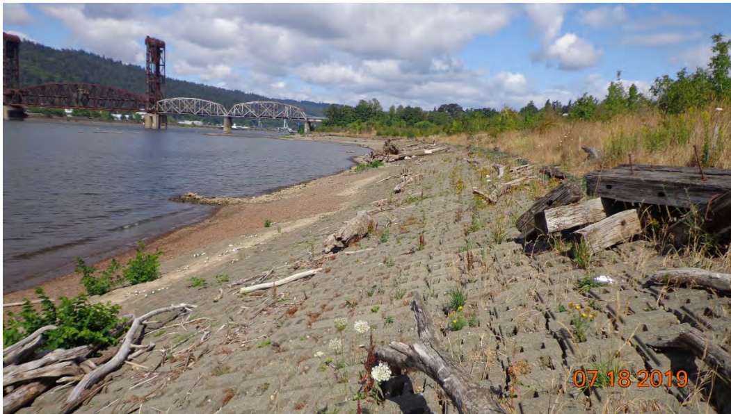
Photo 3 –View of riparian area shoreline with gravel and ACB coverage.
