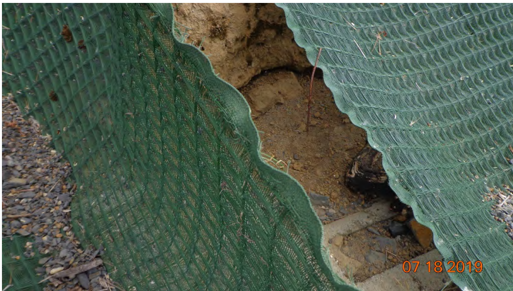
Photo 4 –View of small erosional pocket between seam of TRM.
