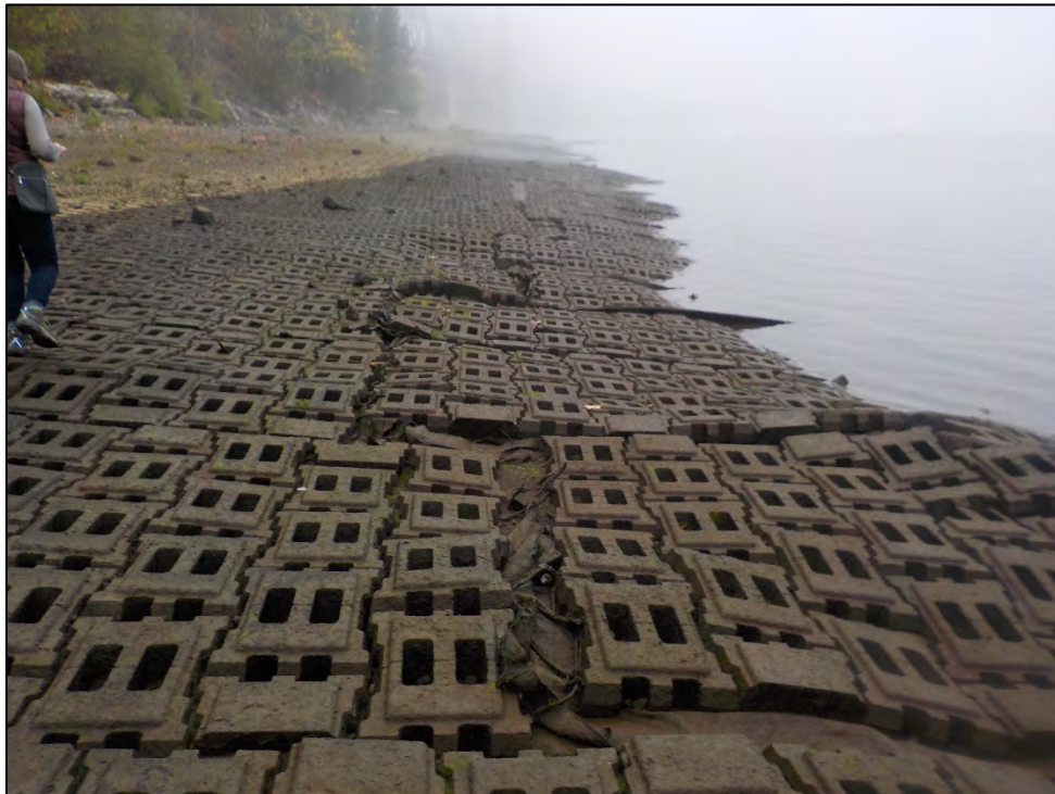
Photograph 11: Separation of ACB mats results in voids, October 2018.
