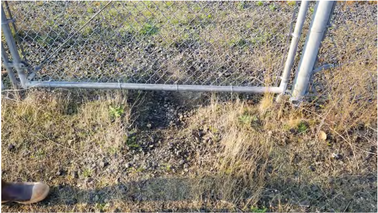
Photograph 5: Burrow underneath fence gate along southwest perimeter of site.
