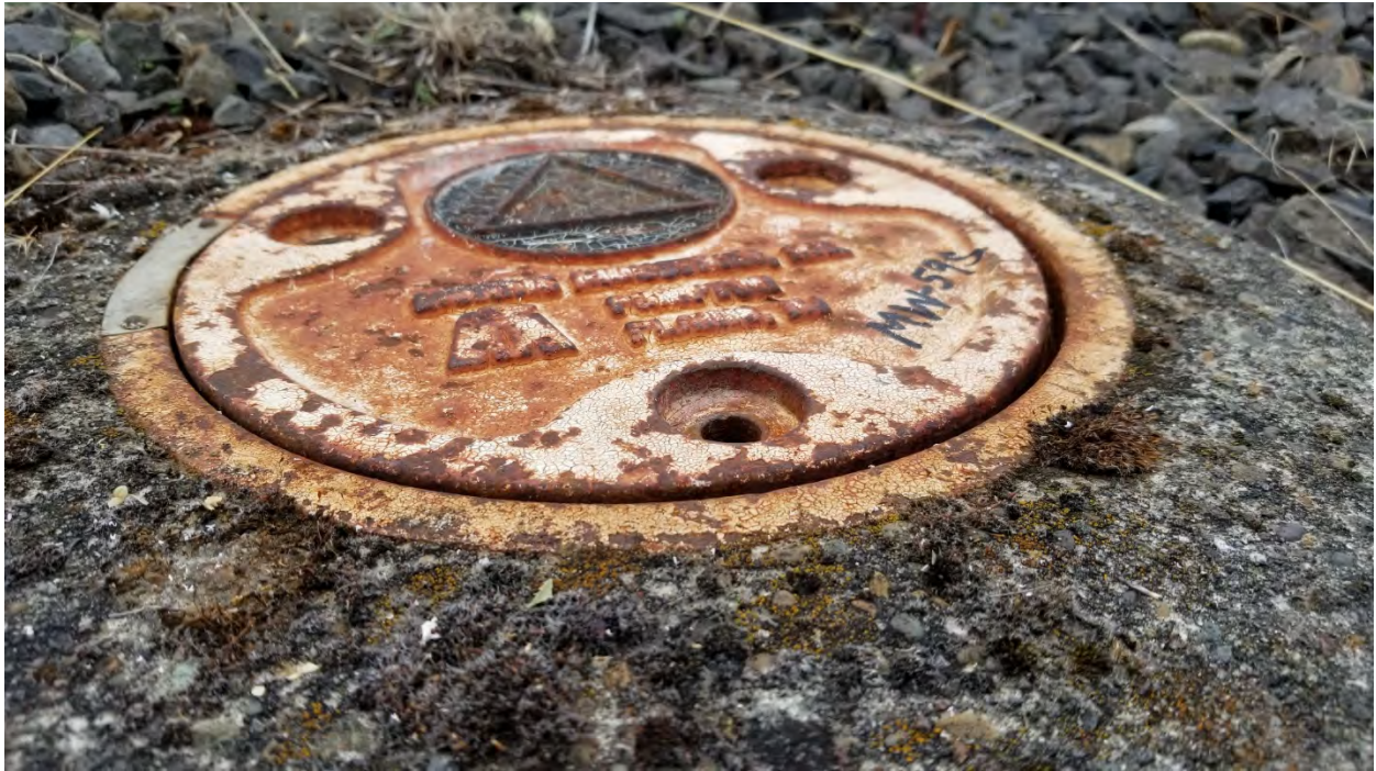
Photo 11: Well lid sitting correctly in well box after trimming of MW-59s casing.
