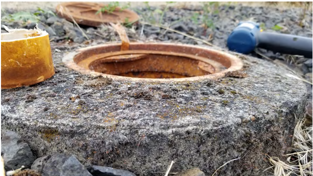
Photo 10: Well casing sitting below the rim of the well box after trimming.
