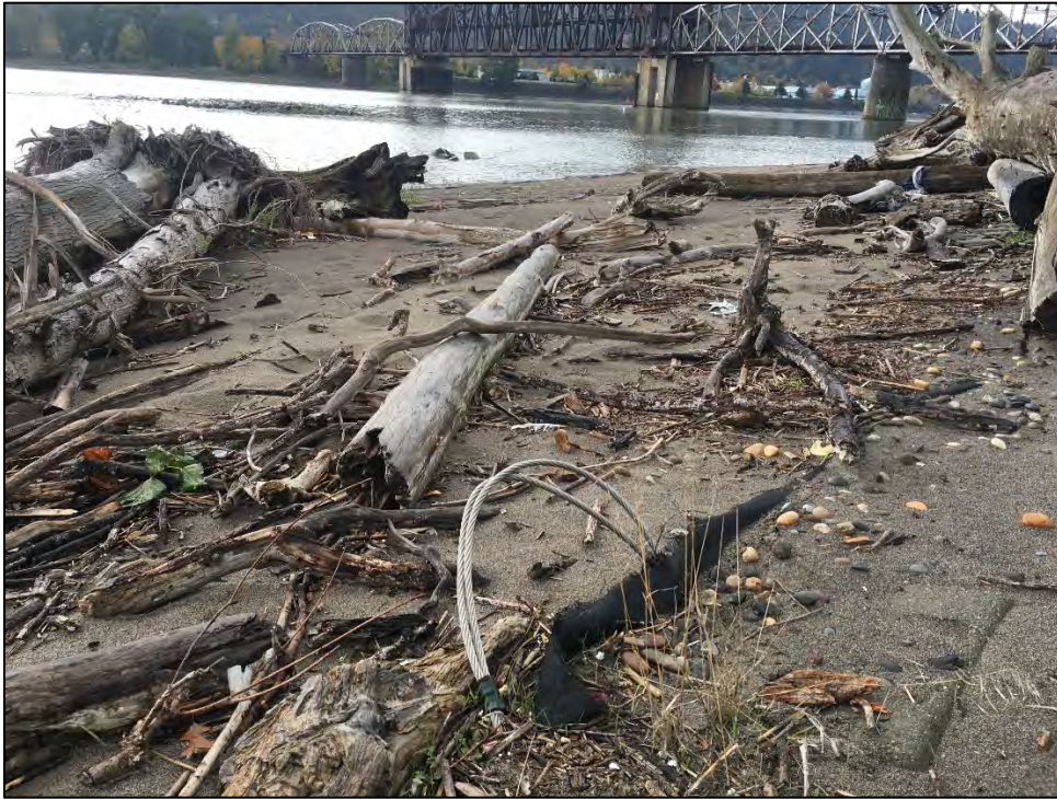
Photograph 1: Cable loops from ACB mats that were cut during maintenance activities to remove trip hazard, October 2016.
