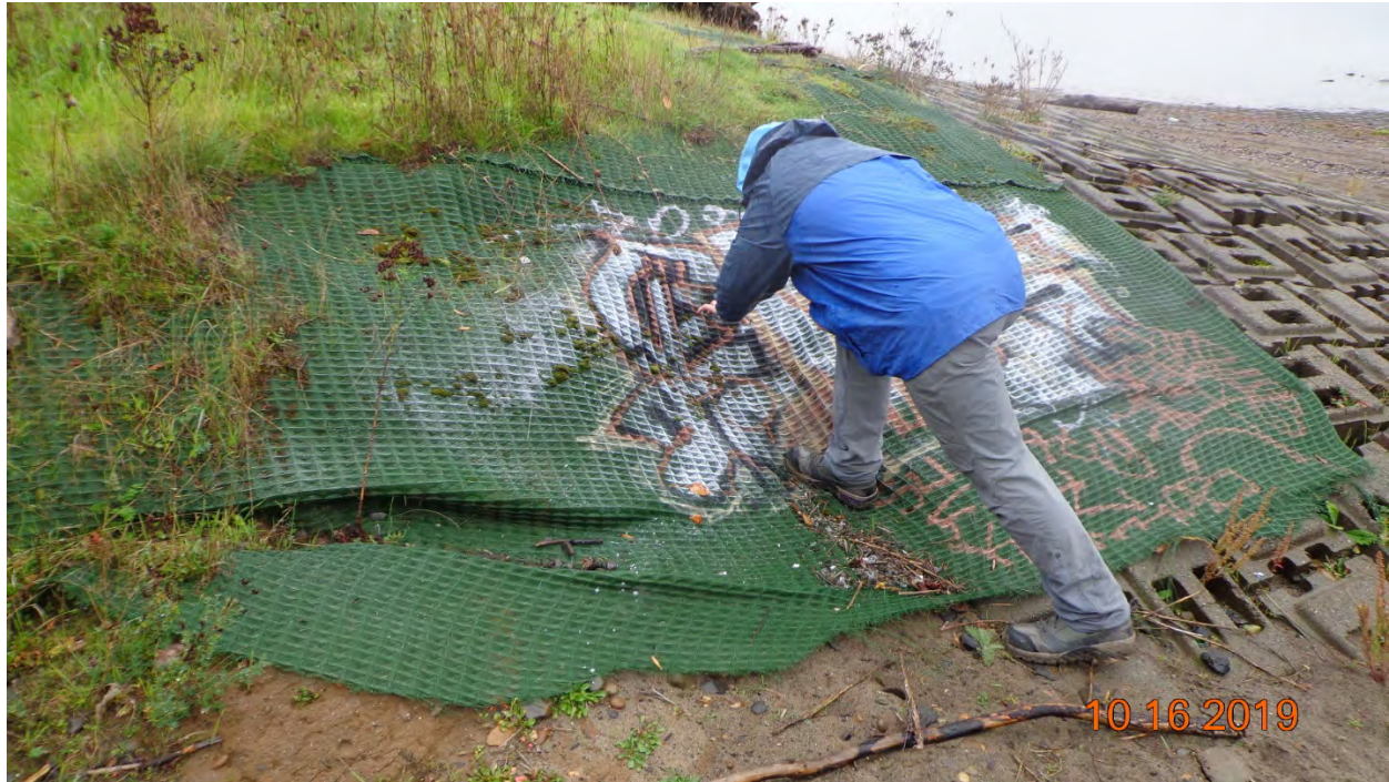
Photo 1: TRM at northern end of riparian area displaying signs of sagging.
