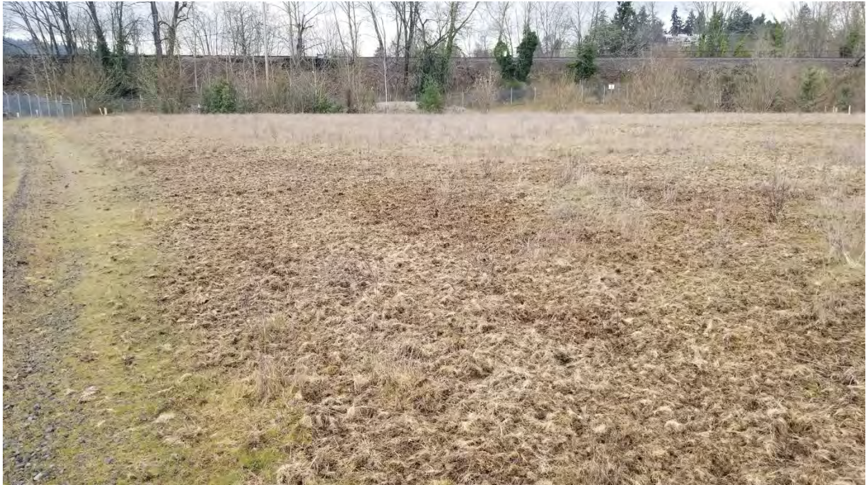
Photograph 7: Impermeable cap surface vegetation following crow foraging activities.
