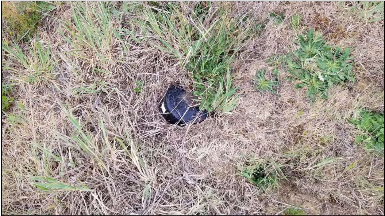
Photograph 5: PVC riser and cap protruding through the soil cap and presumed to be a storm sewer cleanout.
