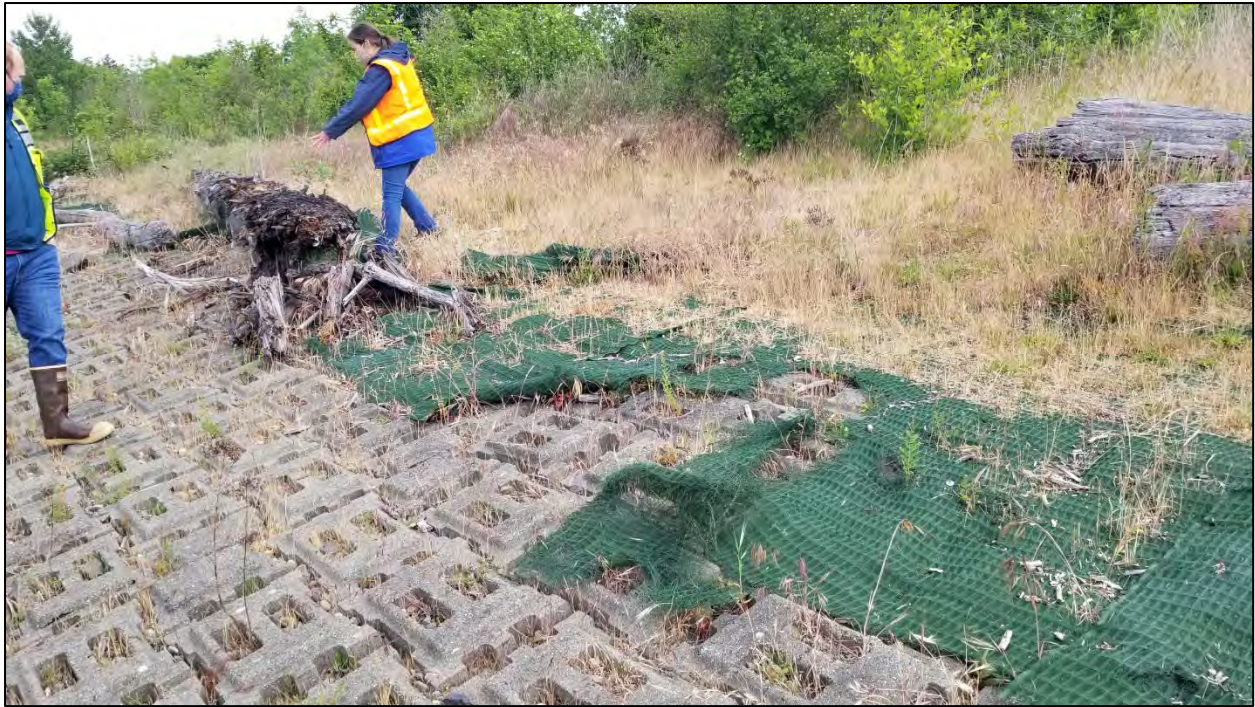
Photograph 3: Loose or torn section of TRM that requires repairs. View facing north.
