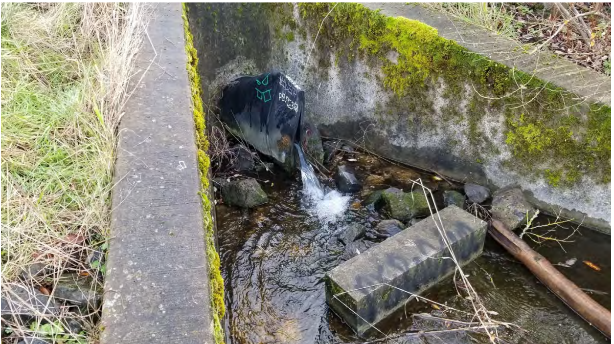
Photograph 2: Stormwater outfall discharge at an estimated 5-10 gallons per minute.
