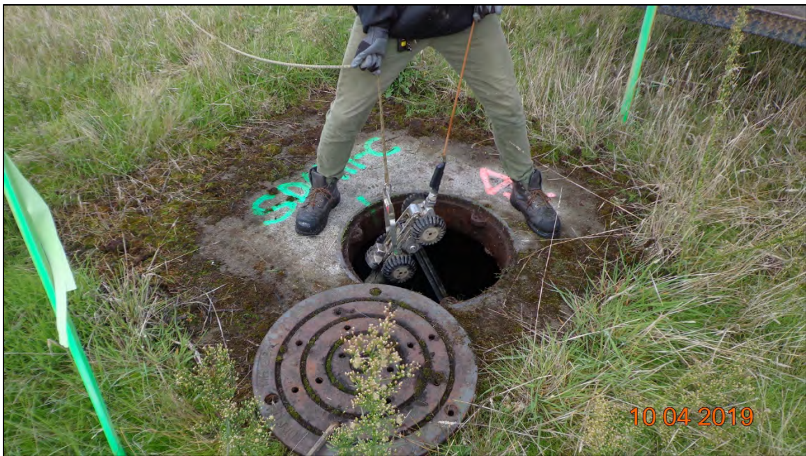
Photograph 14: Storm sewer video inspection using a remote crawler during subsidence monitoring evaluation, October 2019.
