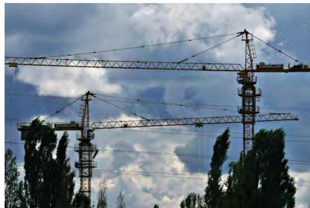
Figure 3: Cranes are especially vulnerable to lightning.
