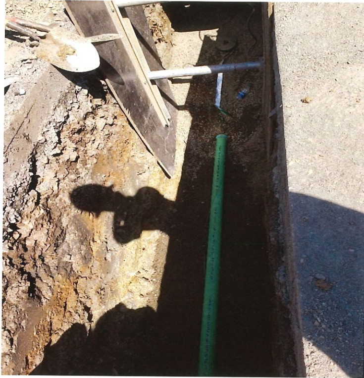
View to the East, \frac{3}{4} -0 gravel, green tracer wire and reflective tape.
