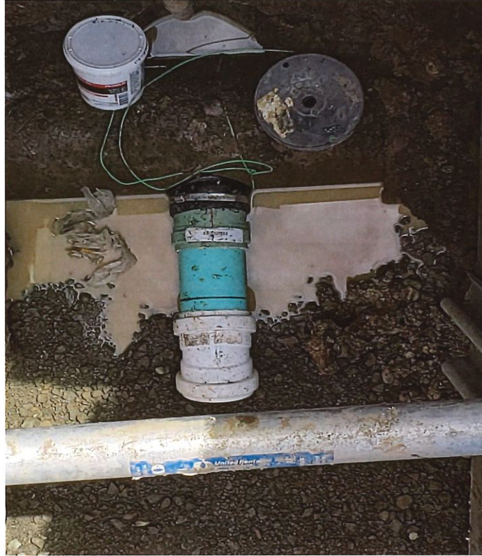
View to the East Inserta Tee connection to sewer main line.
