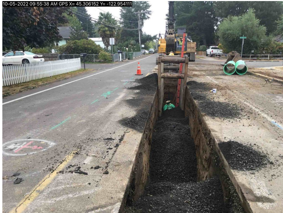
Storm Drain Installation on Elliott Rd
