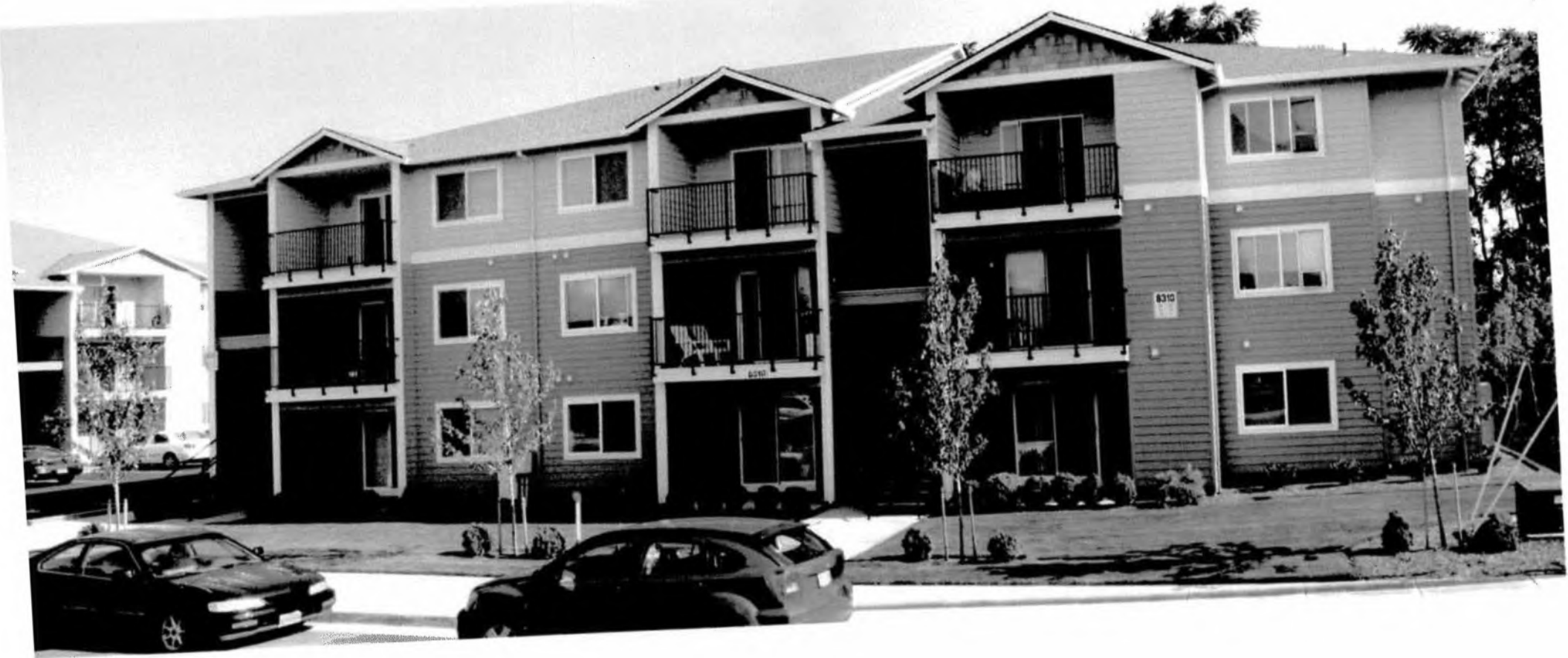
18 UNITS 8310 S.E. RHINE PORTLAND
