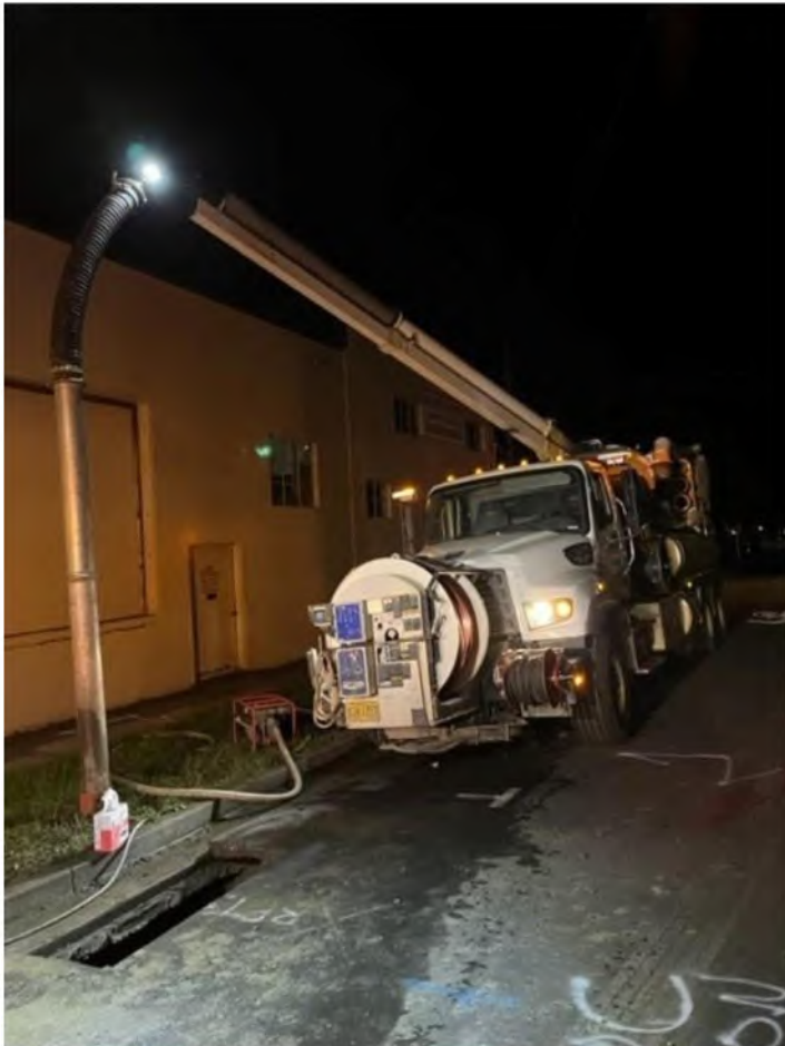
Late night water leak repair Meridian and 2 nd St.
