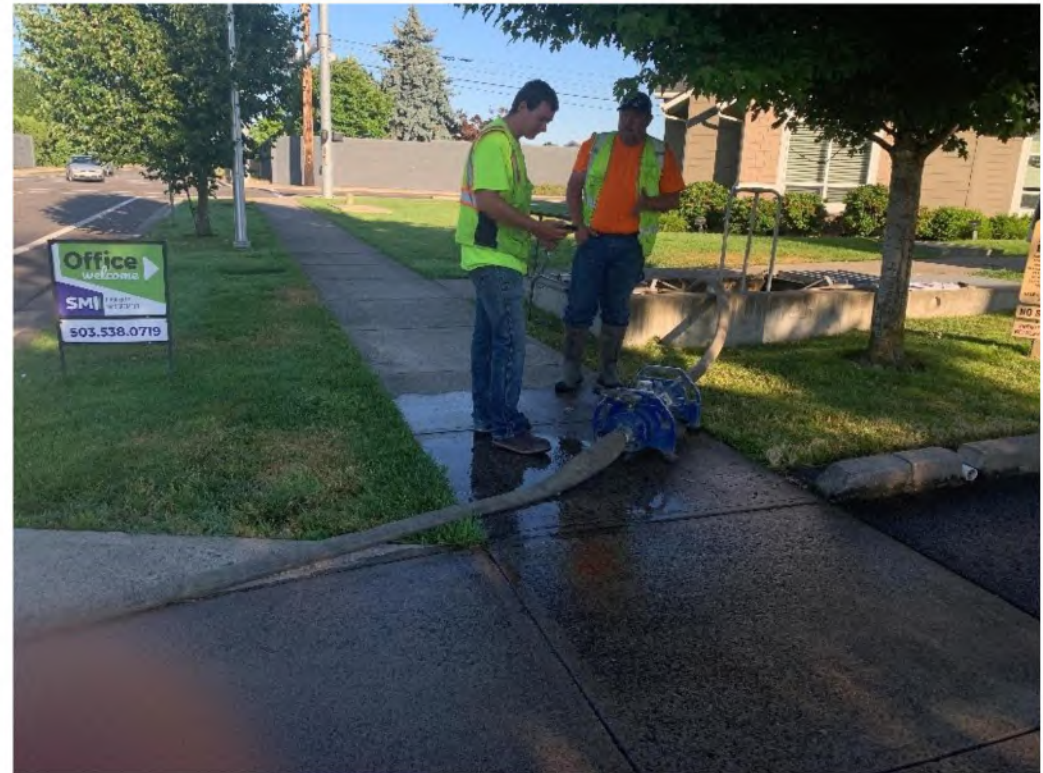
Crews conducting large meter testing
