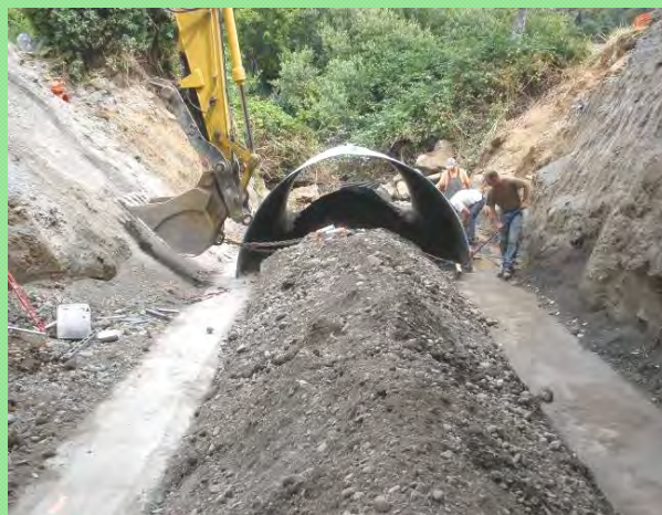
The new culvert features boulders and bottom of natural stream bed material.
