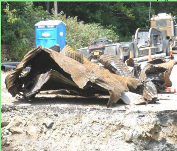
The old culverts were rusty and partly filled with concrete, badly in need of upgrading and replacement.
