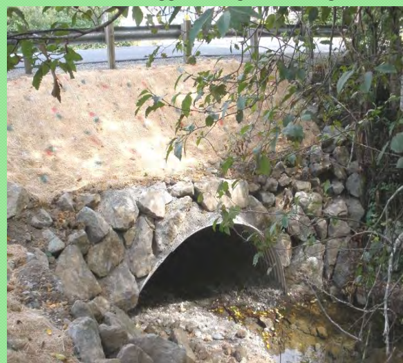
The new Riley Creek inlet. Replacing the culvert at Quarry Road has opened fish access to an additional 0.35 miles of habitat.
