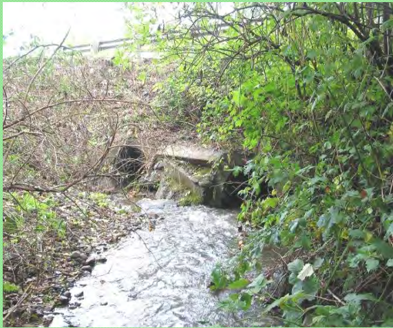
The old Riley Creek culvert inlet at Quarry Road. The old culverts were undersized and contributed to erosion and degraded habitat on the creek.
