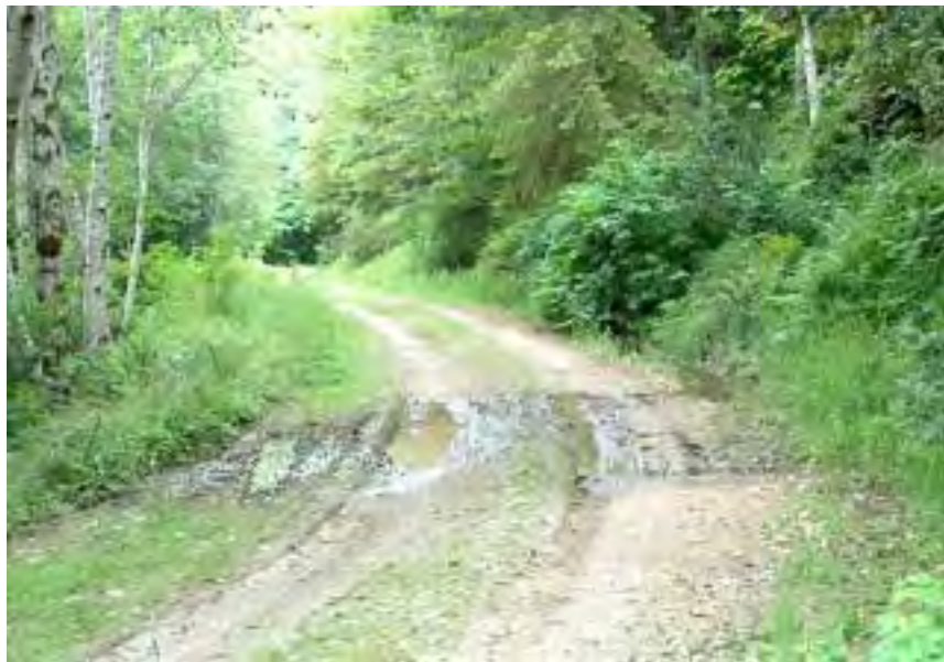
While this does not look like a problem on the surface, this undrained spring was saturating the slope and creating a rotational failure. A cross drain was added. —Photo and article by Matt Swanson
