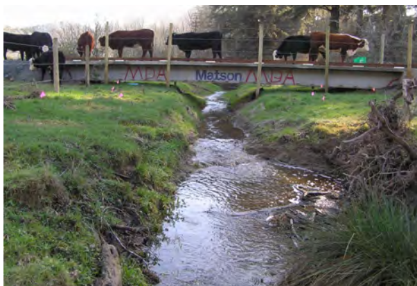
A sea container bridge with concrete deck land to the Winchuck estuary.
