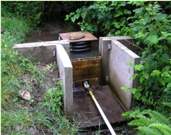
A simple, solid offstream water system intake.
