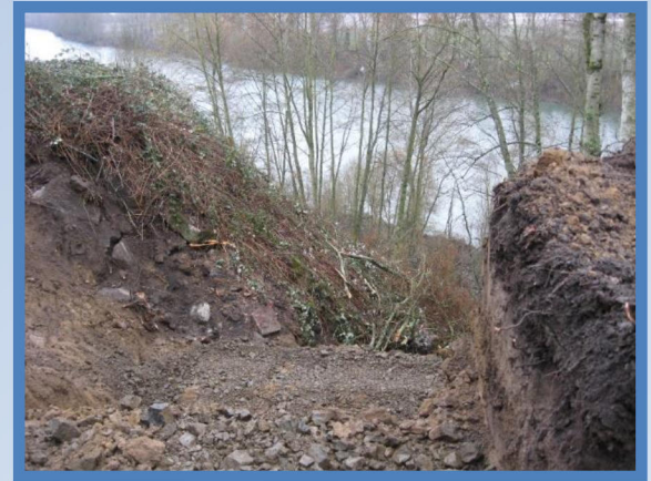
2009 Bank Failure Repairs
