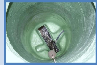
Manhole Lining (complete)
