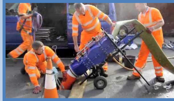
Fiberglass Pipe Lining
