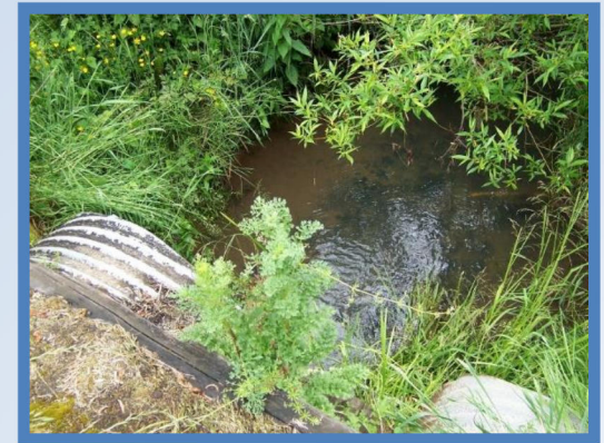
Villa Rd. Hess Creek Culverts
