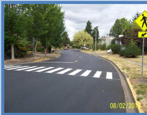
2013 Vitoria Way Thin Lift Overlay
