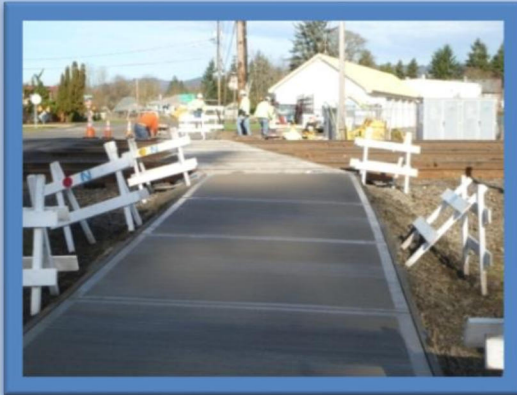
New sidewalk at Railroad Crossing
