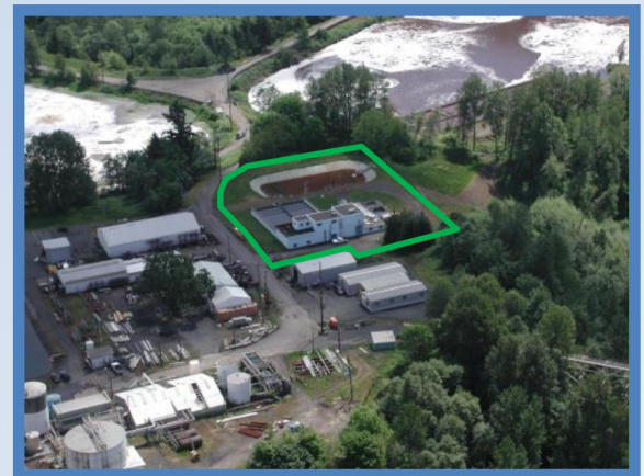
Existing Water Treatment Plant Aerial
