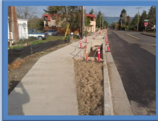
New sidewalk at Deskins Street & College Street
