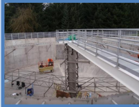
Clarifier #4 During Construction
