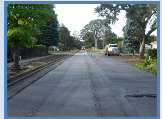
2014 Villa Road Reconstruction
