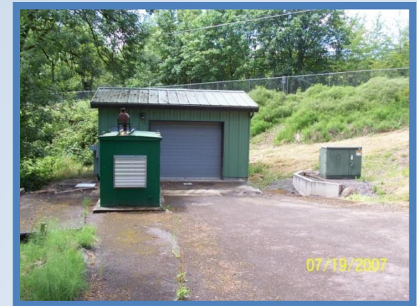
Dayton Pump Station Site
