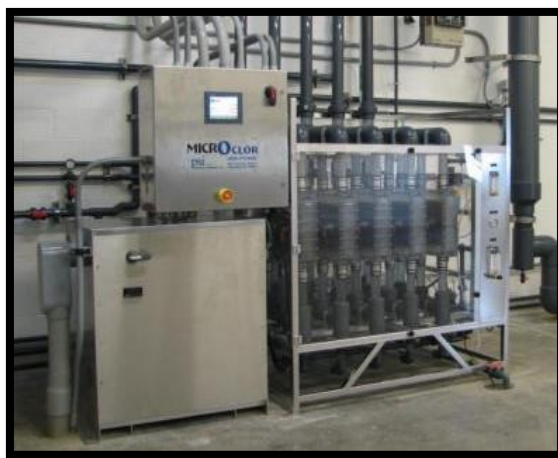
FIGURE 2 PROPOSED WATER TREATMENT PLANT SODIUM HYPOCHLORITE GENERATOR
