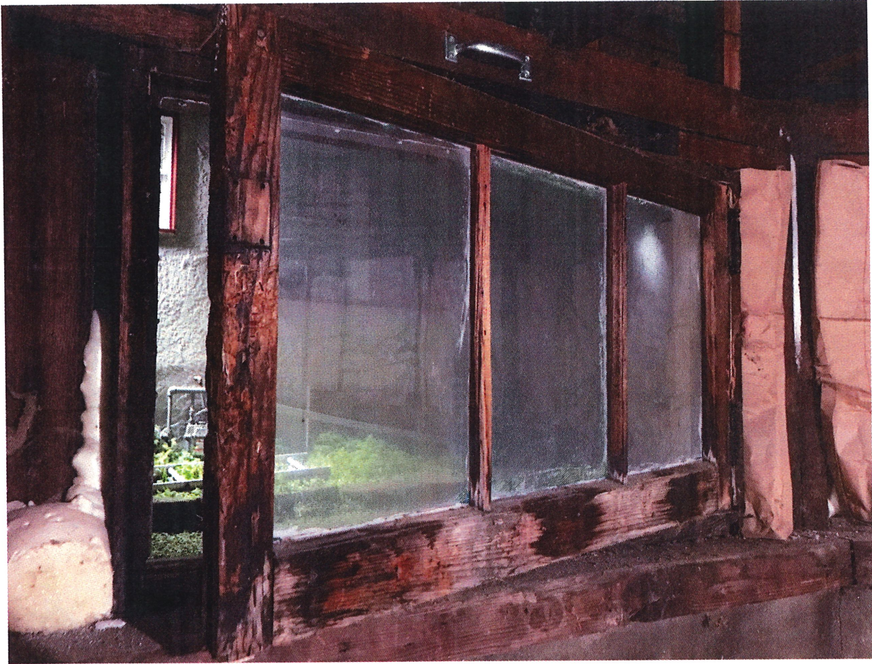
All windows so deteriorated that they are literally rotting off the hinges.
