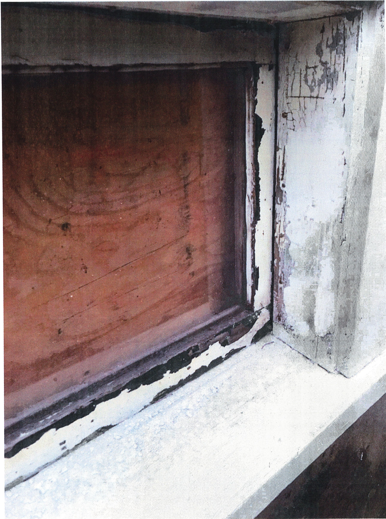
All windows dry rotted with decades of deterioration due to failed caulking.
