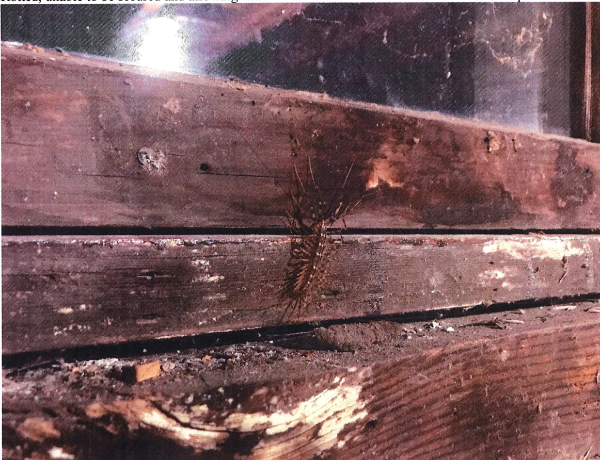
Rotted, unable to be secured and allowing water to encroach on the structure we all seek to preserve.
