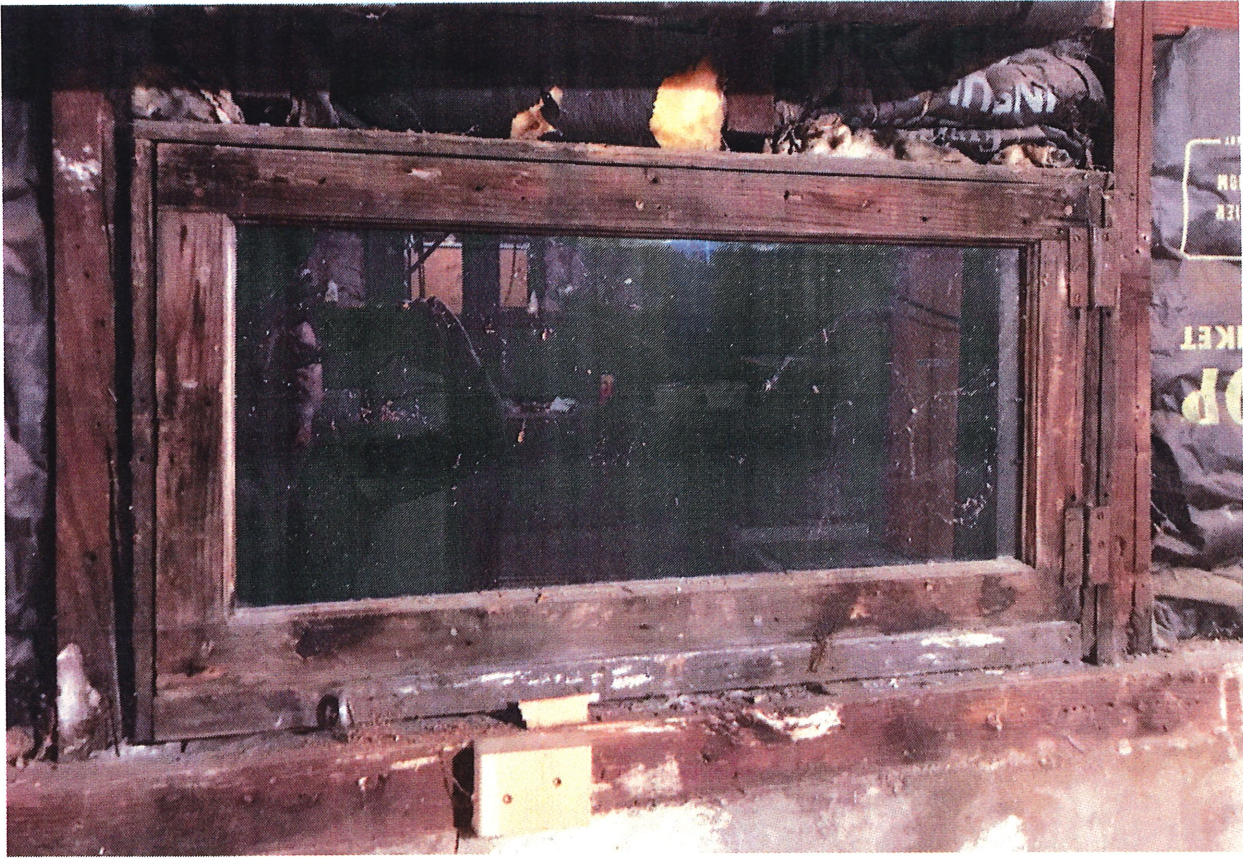
Rotted, unable to be secured and allowing water to encroach on the structure we all seek to preserve.
