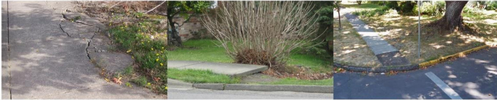
Cracks/Not-level
