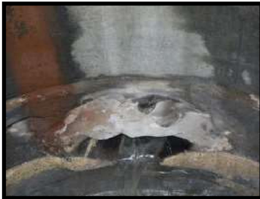
FIGURE 18 INFLOW & INFILTRATION AT THE FERNWOOD & CREEKSIE LIFT STATION
