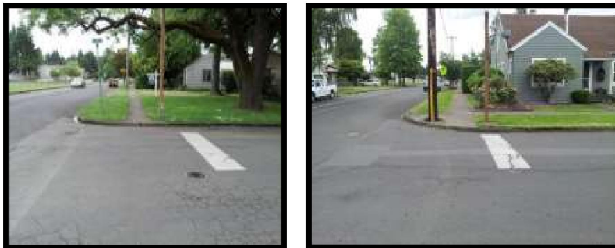
FIGURE 7 CURB RAMP NEEDED
