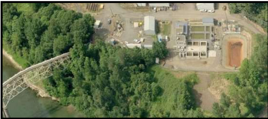
FIGURE 43 WATER TREATMENT FACILITY SEISMIC RESILIENCY
