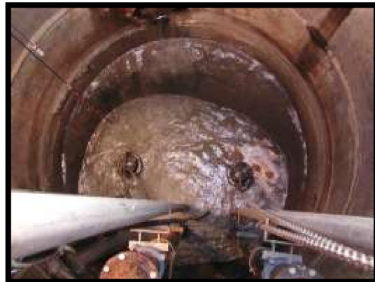
FIGURE 18 INFLOW & INFILTRATION AT THE FERNWOOD & CREEKSIE LIFT STATION
