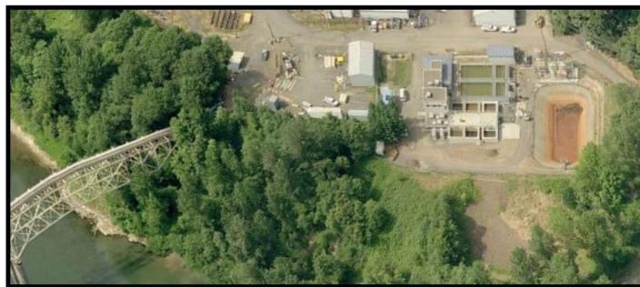
Figure 1: Water Treatment Plant and Water Line Transmission Bridge
