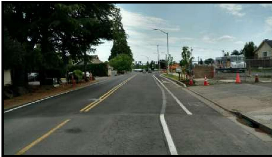
FIGURE 4 LOOKING SOUTH ON ELLIOTT ROAD
