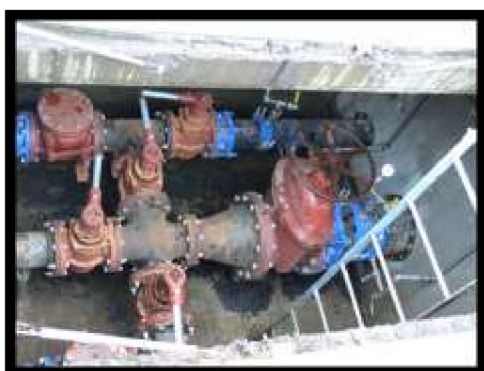
FIGURE 30 FERNWOOD VALVE VAULT
