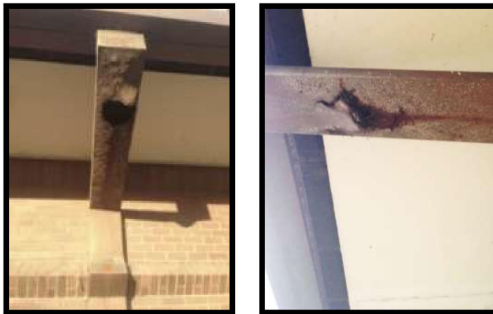
FIGURE 23 ROOF MAINTENANCE AT WASTEWATER TREATMENT PLANT
