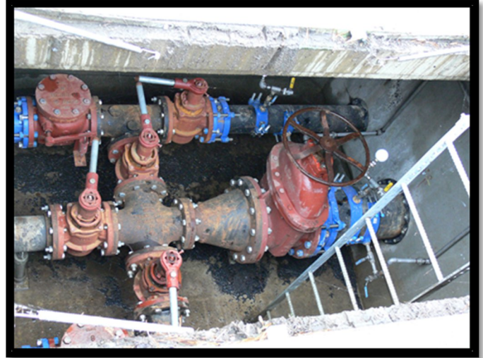
FIGURE 13 FERNWOOD VALVE VAULT
