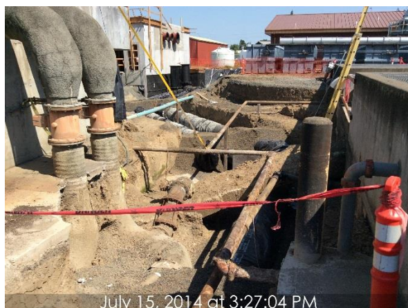
Figure 2: Underground Piping
