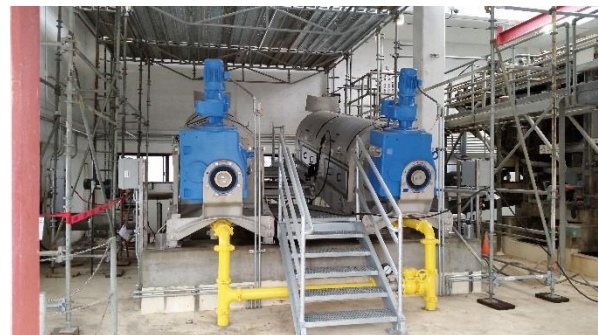
Figure 3: Screw Presses Installed
