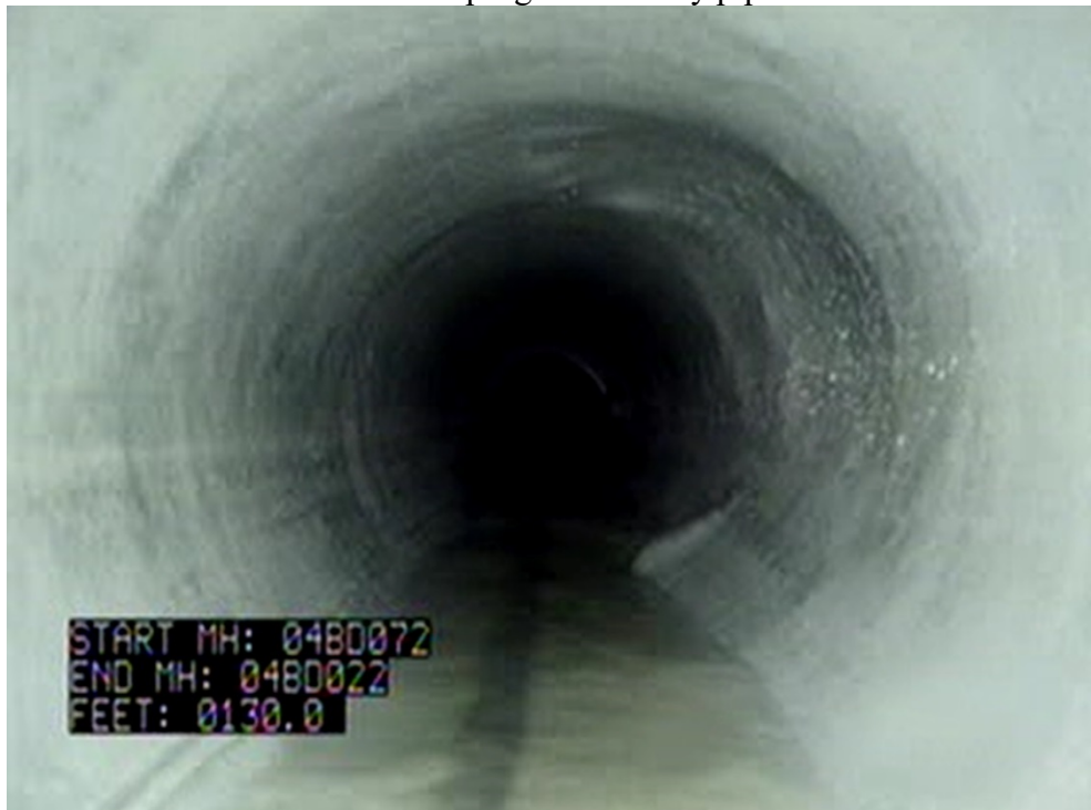
Same location after pipe lining
