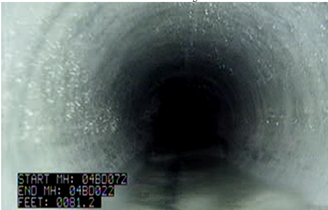
Same location after pipe lining
