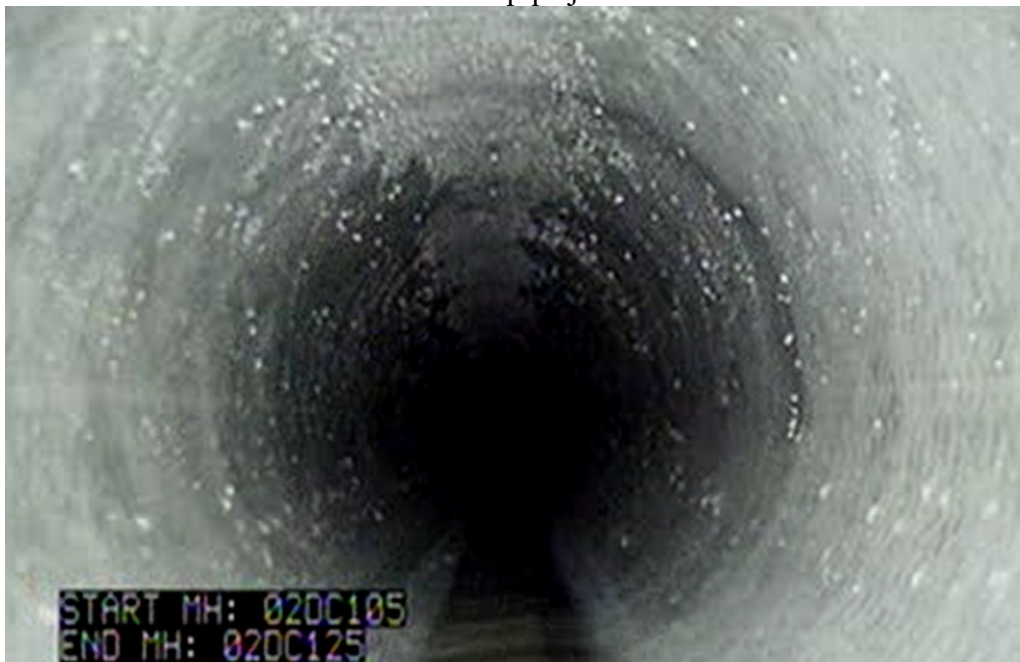
Same location after pipe lining
