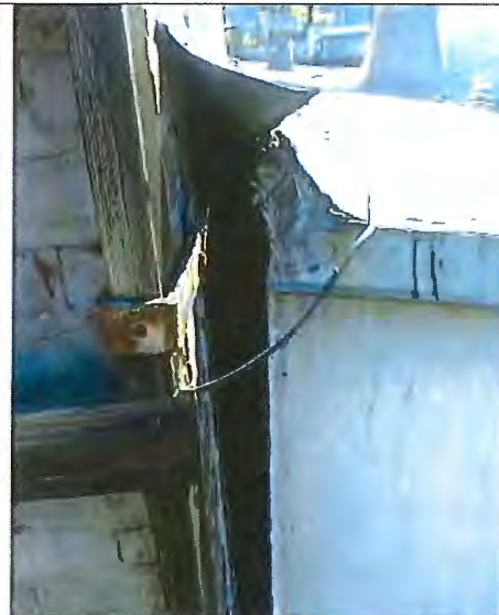
Separation of roof from horn saloon
