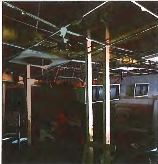
supports to help brace roof from falling
