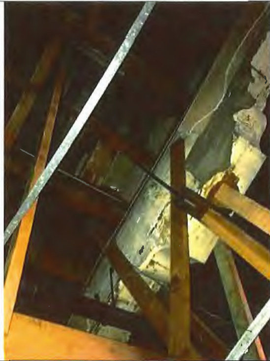
New support to 12 x 12 beam to stop fall
