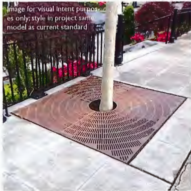
Tree Grates: Color/Finish: Raw Cast Iron Size: 4' wide x 6' length
