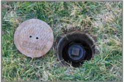
A typical sewer clean out is a pipe with a threaded plug. The plug may or may not be covered as shown.
