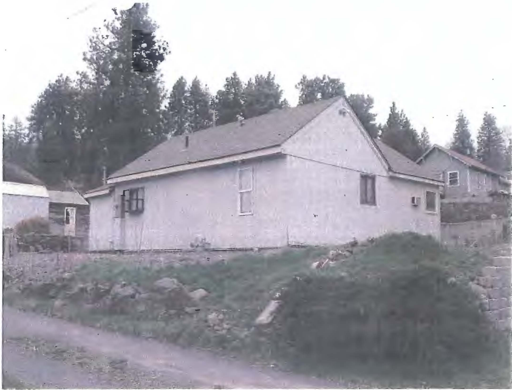
Current Site Condition
