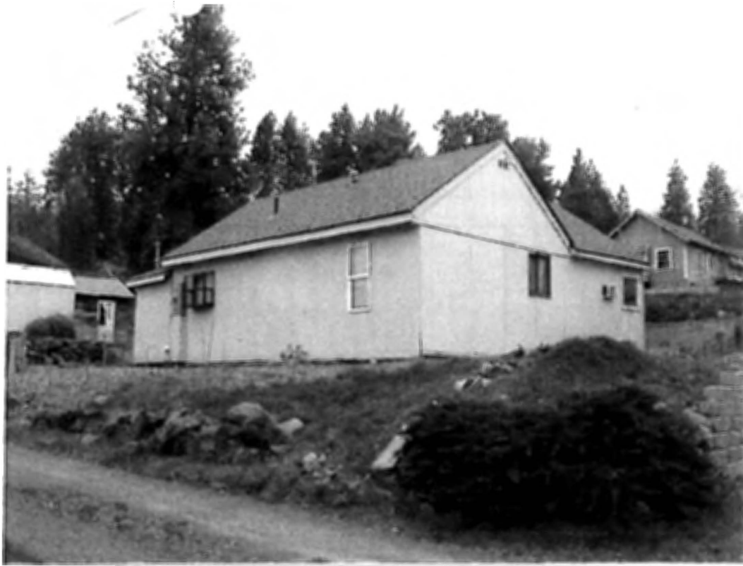
Current Site Condition
