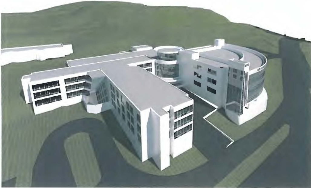
Aerial View from East
