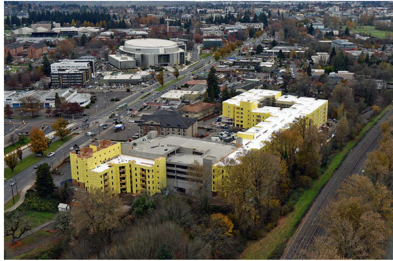
Drone Construction Photo
