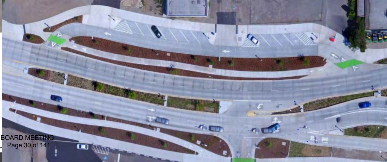
Aerial View of Completed Phase 1
