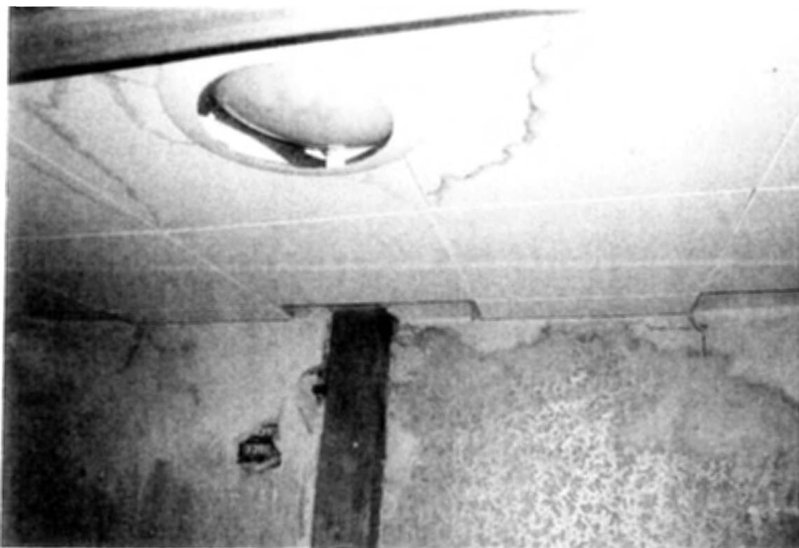
ROOF LEAKS DAMAGING CEILINGS & WALLS
