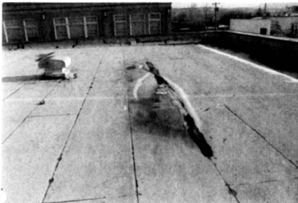
WATER PUDDLES AND DETERIORATES ROOFING
