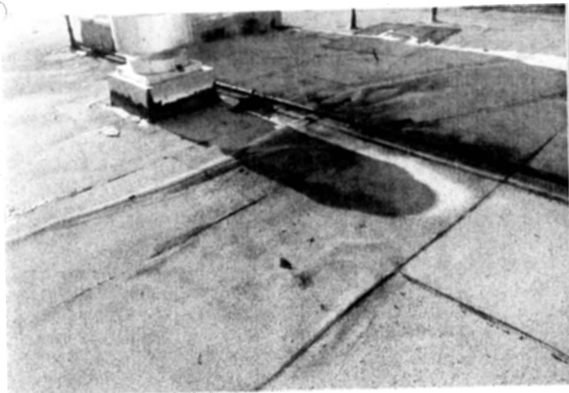
ROOFING BUBBLING AND BUCKLING
