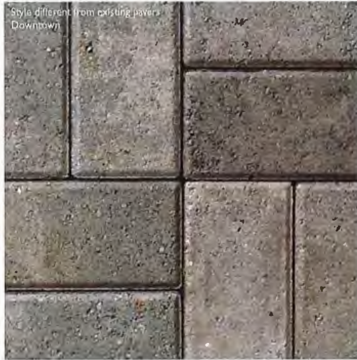
Unit Pavers (Sand Set) Material: Concrete Colors: Range of light grays Pattern: Herringbone with "standard" paver size
