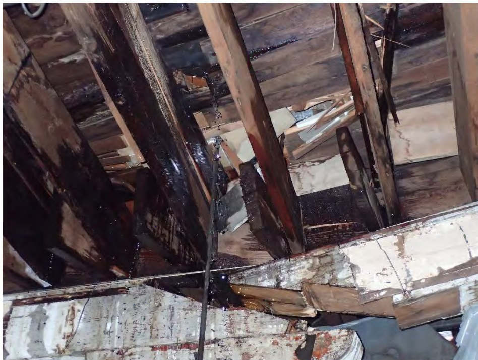
Photo No. 27: Roof structure, water intrusion
