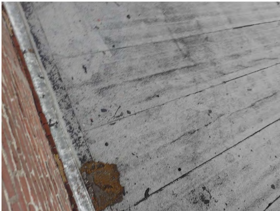
Photo No. 9: Condition of roofing material, visible gap
