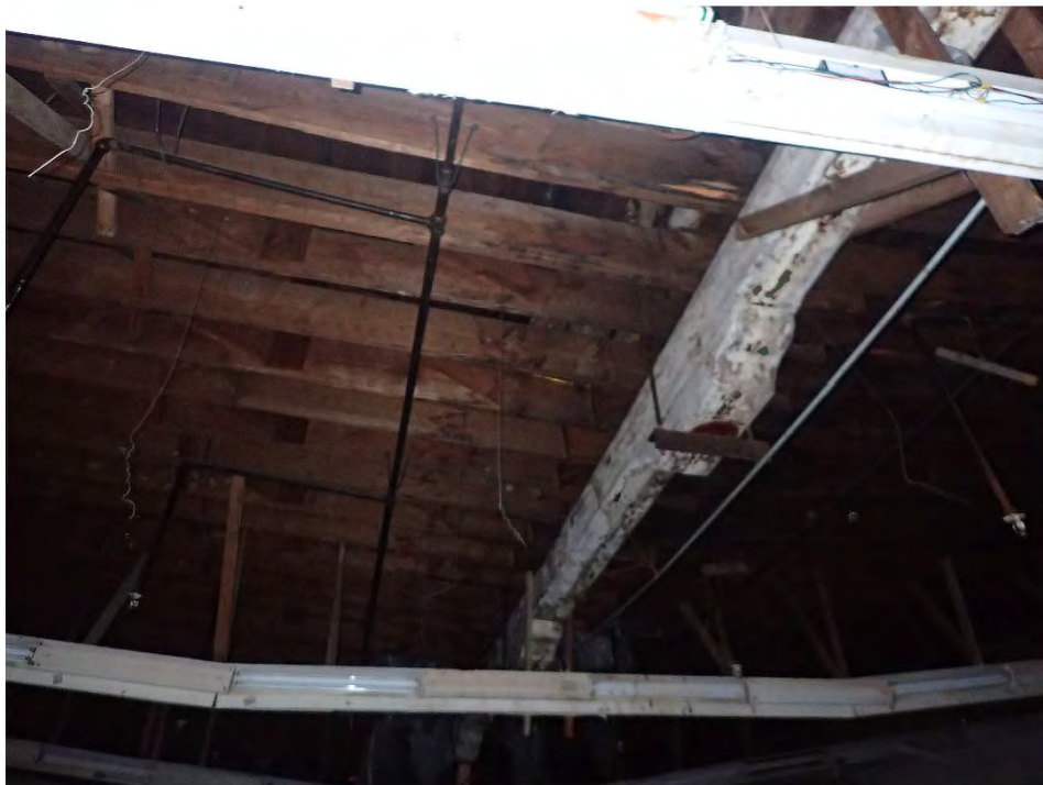
Photo No. 17: View of beam support bracket at previous column locations
