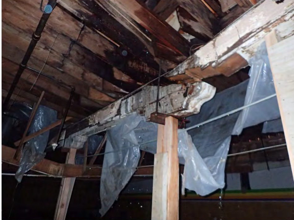
Photo No. 20: Fractured beam and shoring
