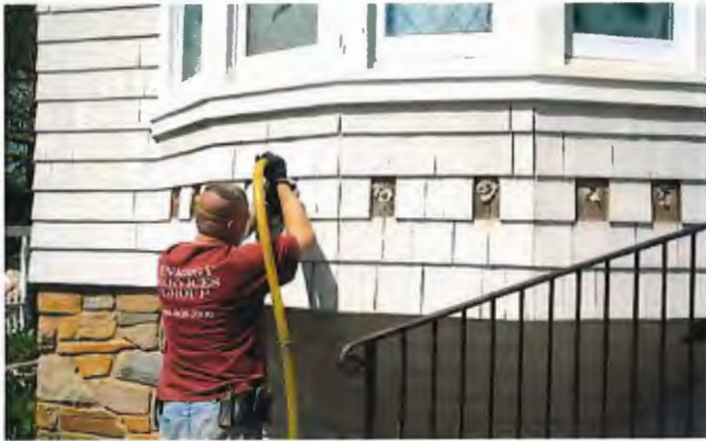
Fig. 18. Dense-packed cellulose insulation is being blown in through holes drilled in the sheathing. Once the operation has been completed, the shingles will be reinstalled. Photo: Edward Minch.
