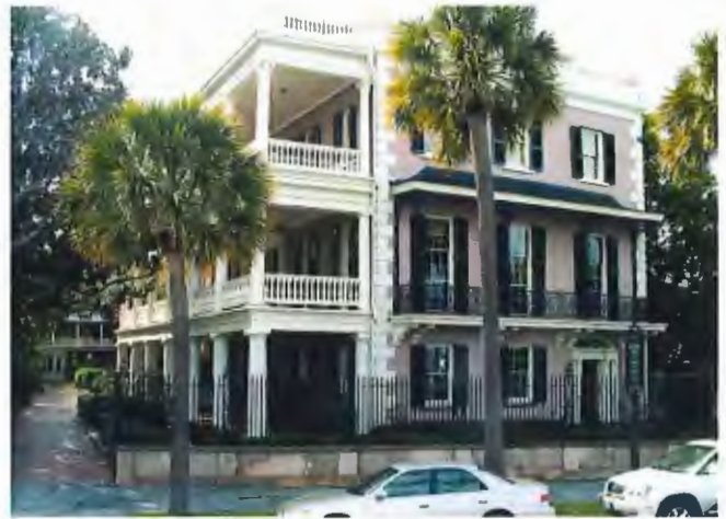
Fig. 5. The side porches of this house in Charleston, SC, shade the large windows and provide outdoor living spaces that take advantage of sea breezes.
