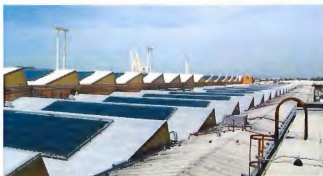
Fig. 23. Solar collectors installed in a compatible manner on low sloping sawtooth monitors. Top Photo: Neil Mishalov, Berkeley, CA.
