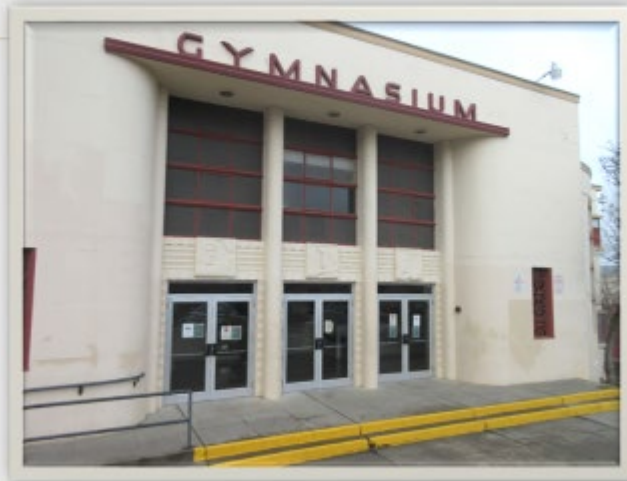
Existing Conditions - The Dalles High School
