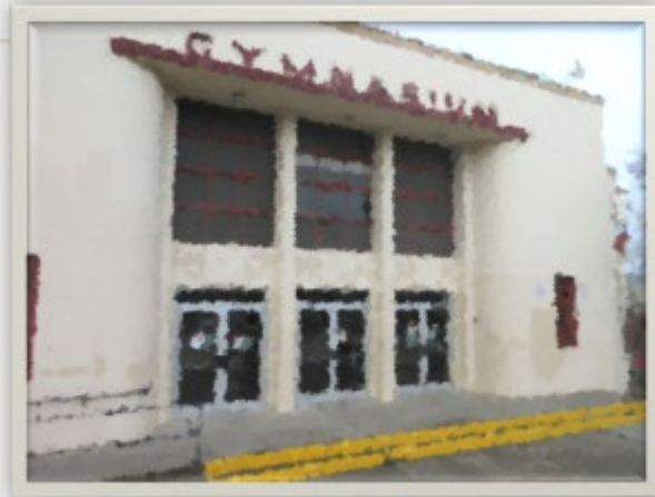
220 East 10th Street - The Dalles High School Gymnasium
