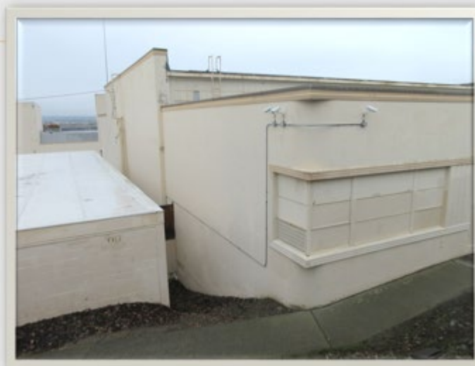
Existing Conditions - The Dalles High School
