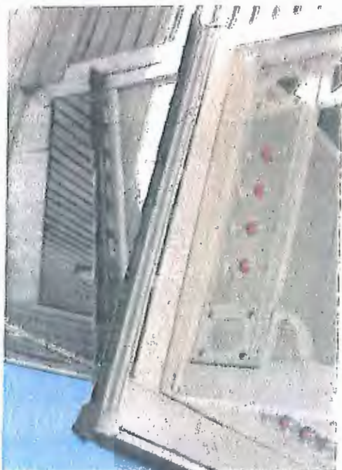
Front roof fascia (front porch) & crown mouldings in need of repair.
