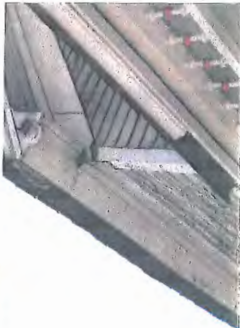
East elevation fascia & crown moulding damage
