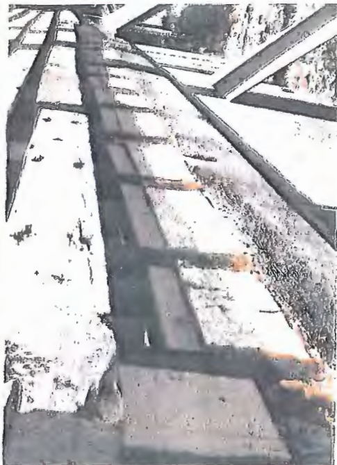
Water table & skirt board needing restoration.
