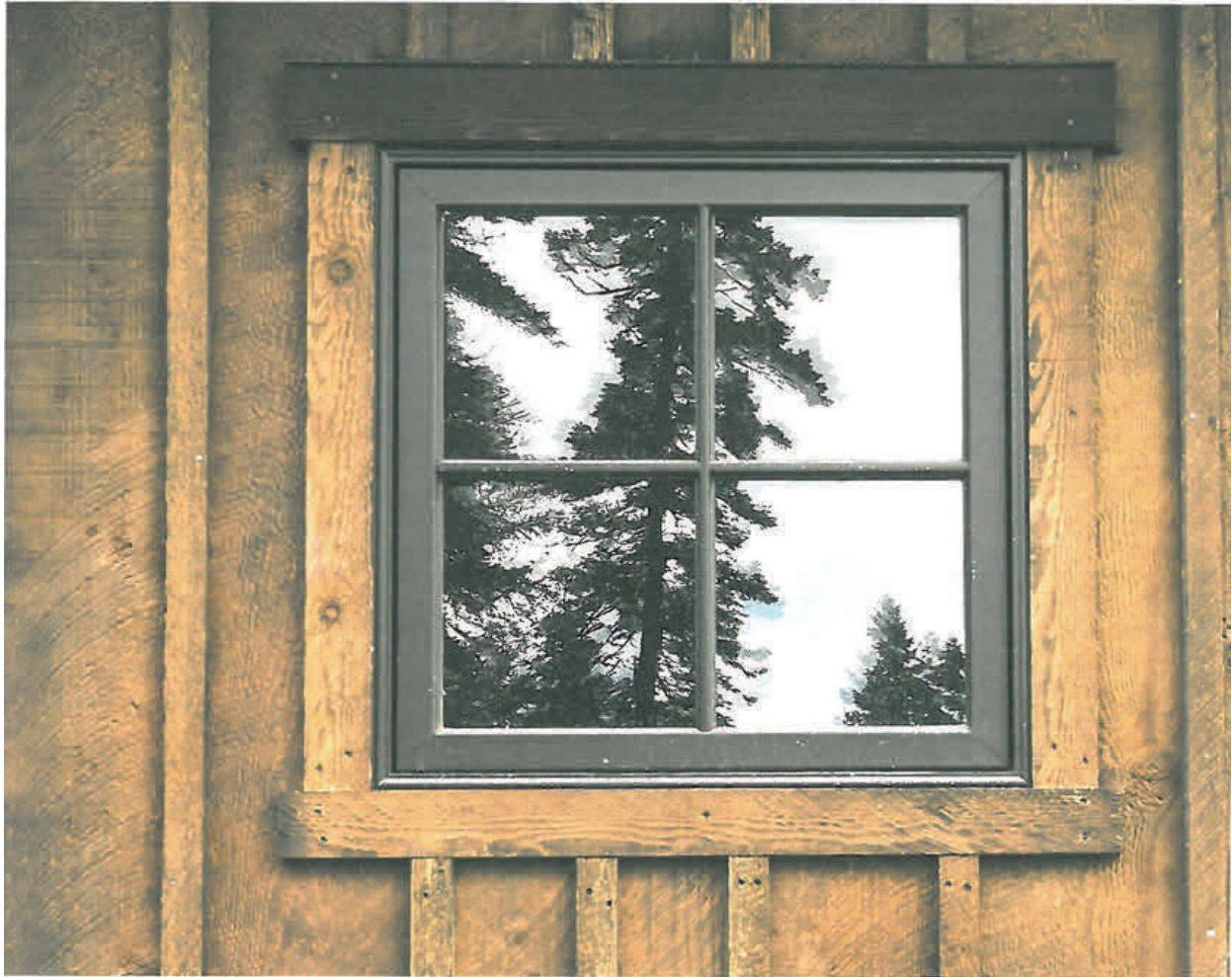
Example of Board & Batten Siding
