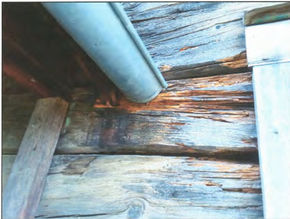
FIGURE 8: DETAIL OF THE ROT ON THE LOGS AT THE PORCH ROOF JUNCTION.
