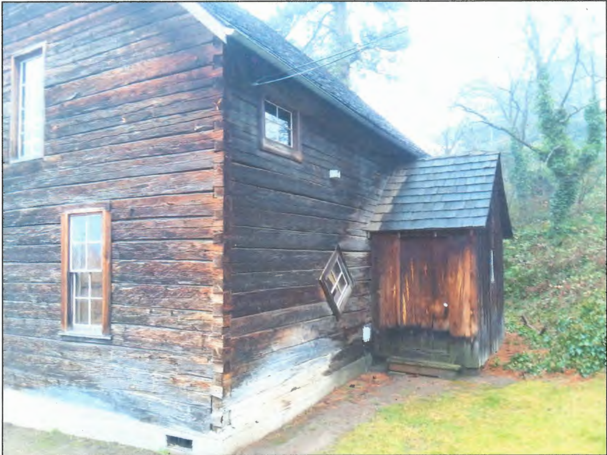
FIGURE 9: ANDERSON HOUSE TODAY, SHOWING THE BACK OF THE HOUSE. NOTE WATER SATURATION OF THE LOWER LOGS BELOW THE DIAMOND WINDOW AND STAINING ON THE PLANK PORCH WALLS.
