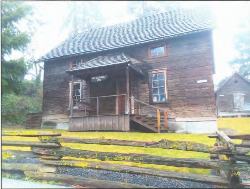
FIGURE 7: ANDERSON HOUSE TODAY, NOTE WATER SATURATION OF THE SILL LOG ON THE LOWER LEFT HAND CORNER AND STAINING AROUND THE PORCH APRON. ALSO, NOTE THE WATER SATURATION OF LOGS AT THE PORCH ROOF EDGE.
