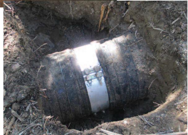
Repair band used to fix leak on the Dog River Pipeline
