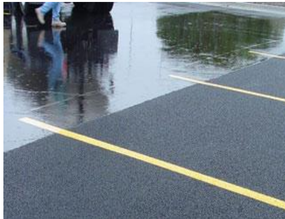
Porous asphalt on right hand side; standard asphalt on left hand side
