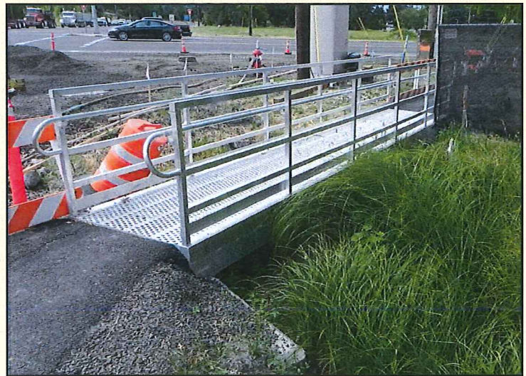
Temporary Pedestrian Bridge use for a TPAR
