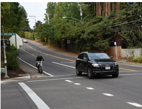
The cross section of Wilamette Street changes several times over its length from downtown to South Eugene.
