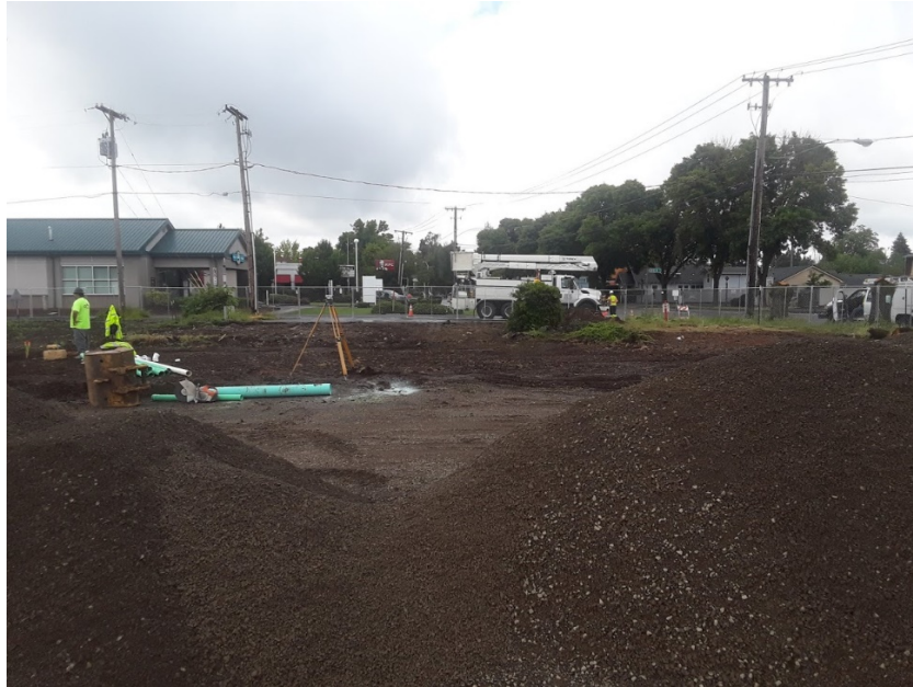
Pictured Above: Post-demolition of the hair salon
