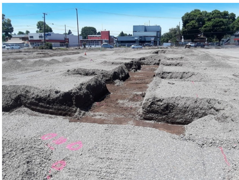
Pictured Above: Footings dug out for bus shelter
