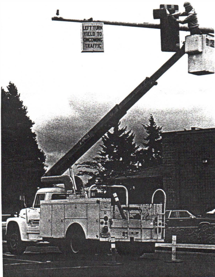
Final touches of signal installation at South Main and Walker Roads.
