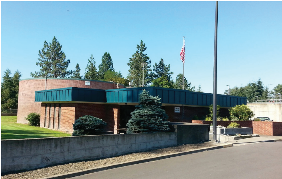
The City of Lebanon Water and Wastewater Treatment Plant (WWTP).
