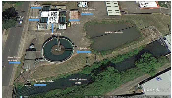
Aerial view of Lebanon WTP.
