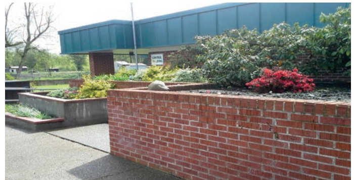
Completed planter area in front of Wastewater administration building.
