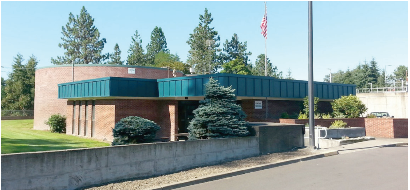
The City of Lebanon Water and Wastewater Treatment facility.
