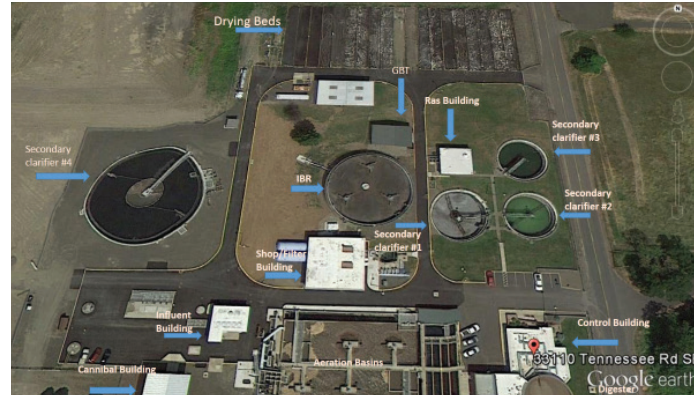
Aerial view of the wastewater treatment facilities.
