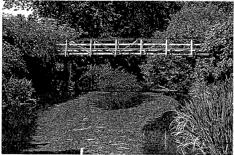
An abandoned overflow pipe will be converted into a walking and biking bridge as part of the Build Lebanon Trails plan.
